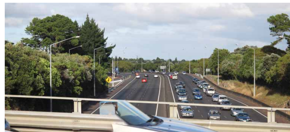
Figure C-6.12: Photo 6-2 View east along SH16 from Carrington Road bridge
