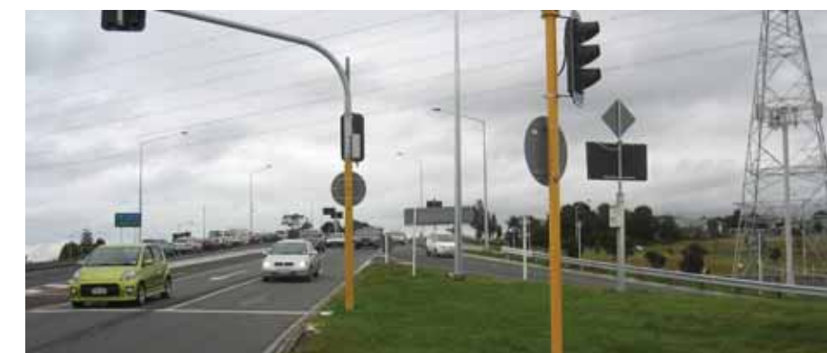
Figure C-1.19: Photo 1-5 Existing view south of overbridge and cloverleaf ramp
