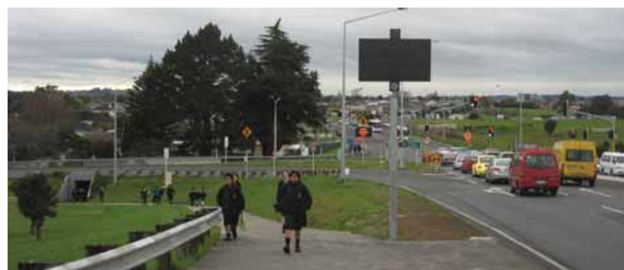
Figure C-1.18: Photo 1-4 View north towards pedestrian underpass and cloverleaf ramp
