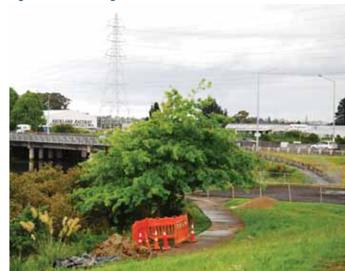
Figure C-1.4: Henderson Creek and connecting off-road path
