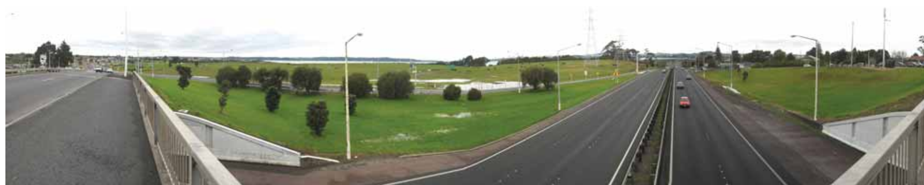
Figure C-1.16: Photo 1-2 Panorama based on existing view from Te Atatu overbridge
