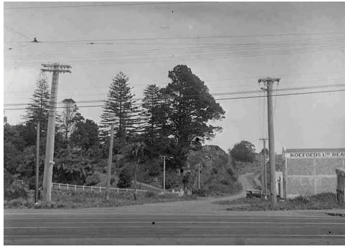
LOOKING WEST FROM BROADWAY ALONG MORTIMER PASS, 1928. SOURCE: AUCKLAND CITY LIBRARIES
