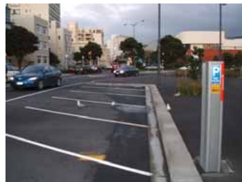
Angle parking bays with central Pay and Display machine
