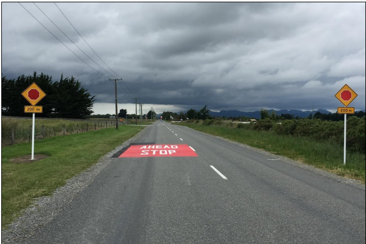
Figure 4-24: “Stop ahead” message marking to draw driver attention to stop control intersection ahead
