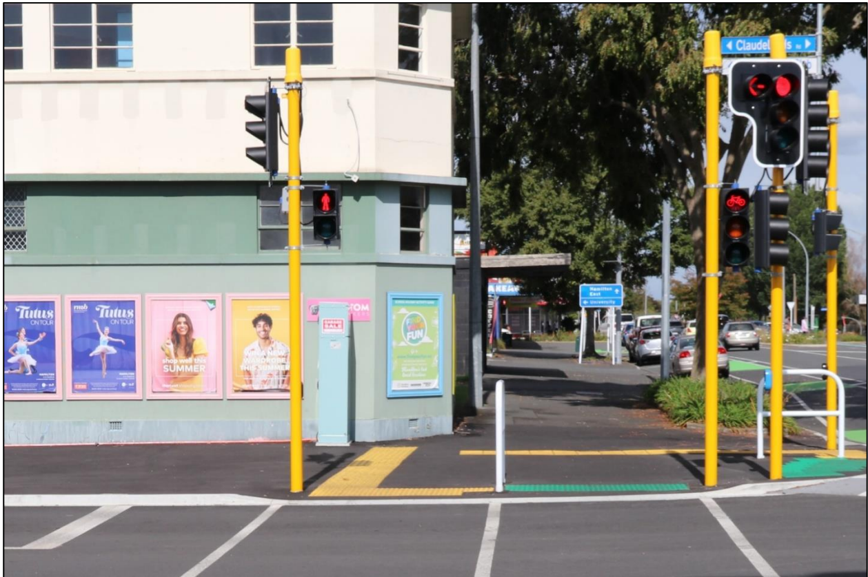
Figure 8-3: Cycle signal display (on right) where cycle path and signalised pedestrian crossing (left) cross the roadway at an intersection
