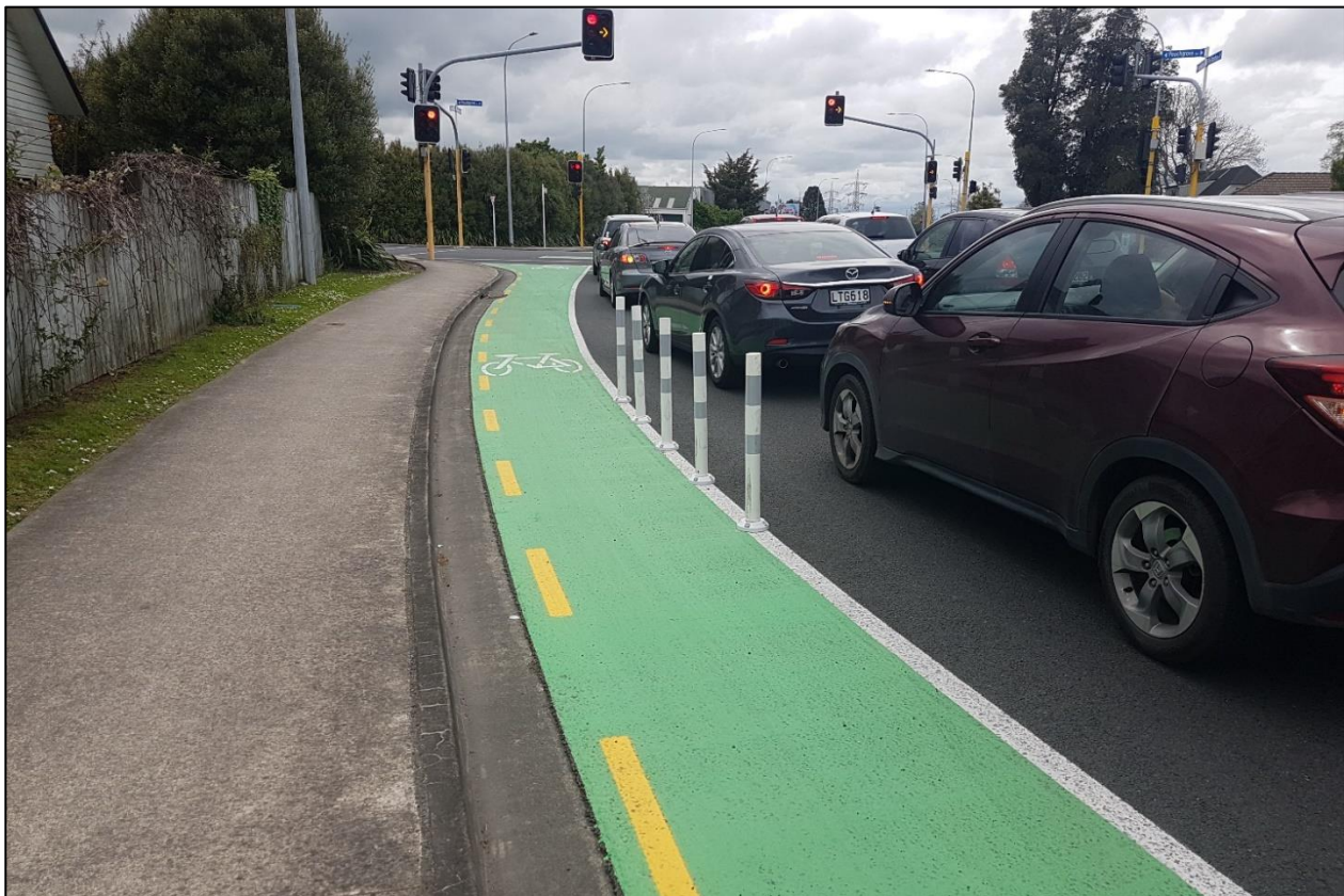
Figure 6-12: Cycle lane leading up to an intersection
