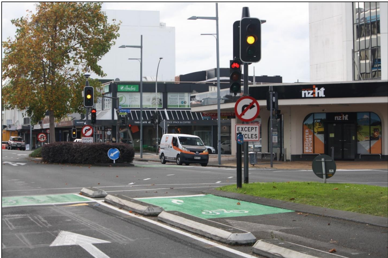
Figure 15-1: Cycle path on approach to signalised intersection where only cyclists are permitted to turn right
