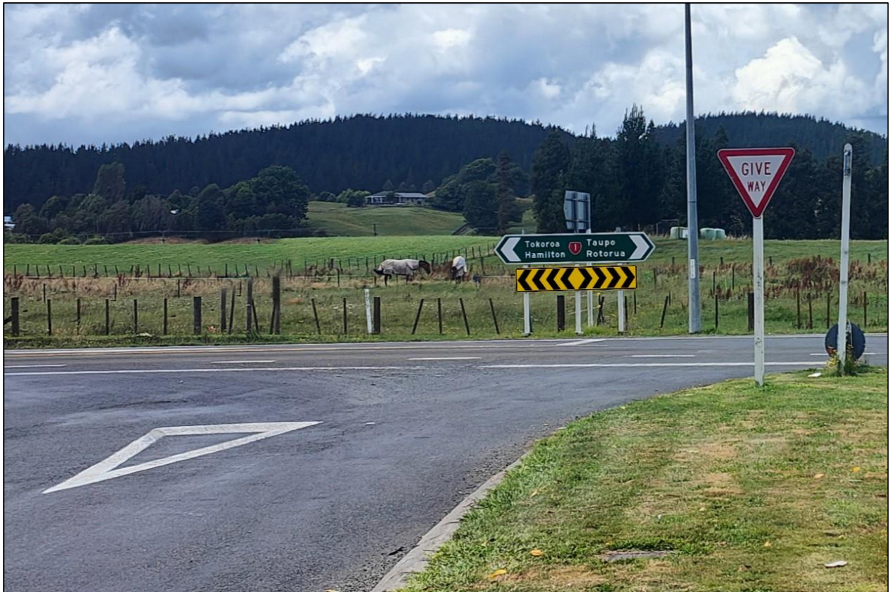
Figure 4-4: Example of Intersection direction sign arrow board two directions (A13-3) at head of intersection, with a W20-1.4 below
