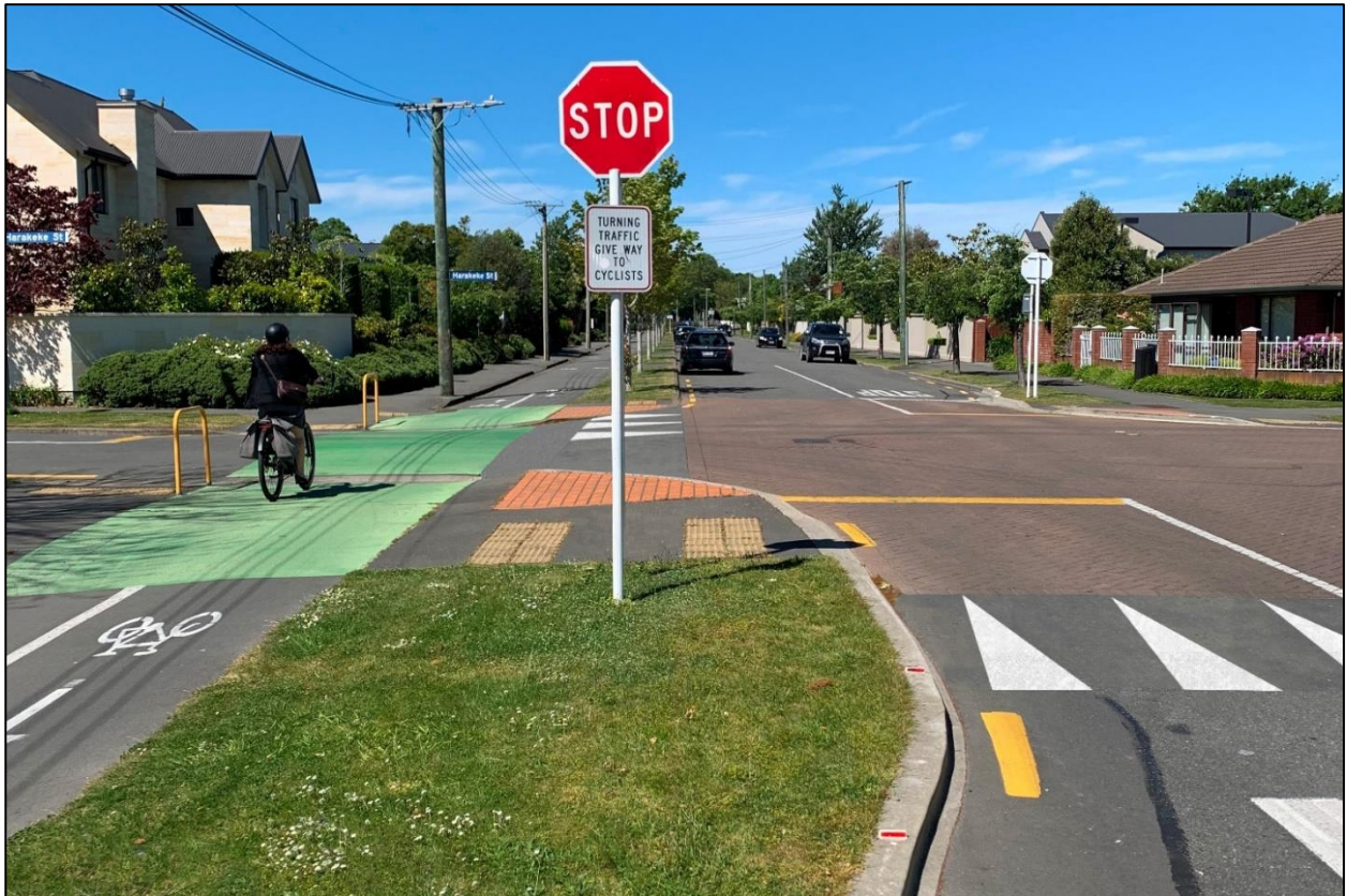
Figure 8-2: Example of an uncontrolled cycle path crossing at four-way stop controlled intersection
