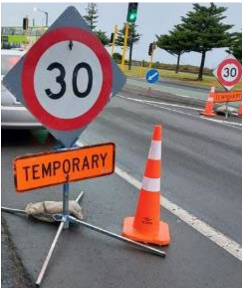
Figure 3.3 Example of temporary speed signs for road works (photo supplied by F. Thomas, April 7 2022)
