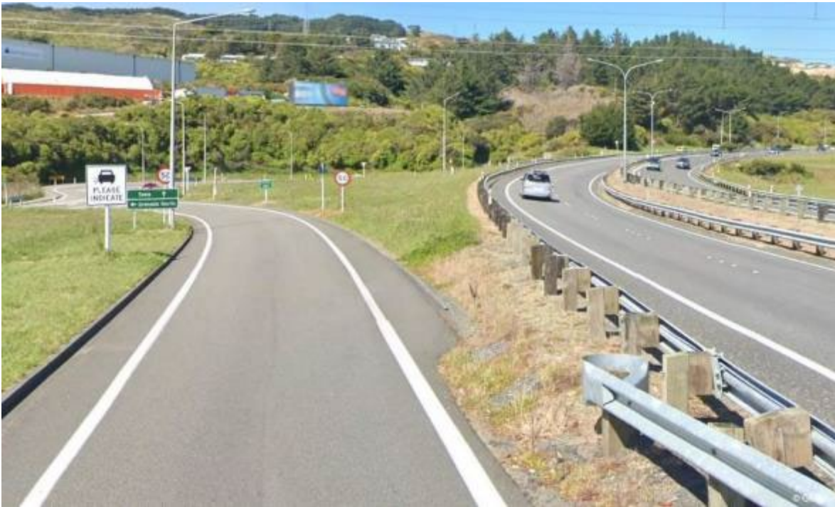
Figure 3.2 Example of adjacent roads where a speed sign could be incorrectly detected if travelling on the road to the right (reprinted from Waka Kotahi NZ Transport Agency Wellington, 2021)
