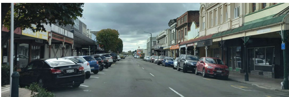
Figure 6.3 Angle parking on one side, parallel parking on the other side (Marton)
