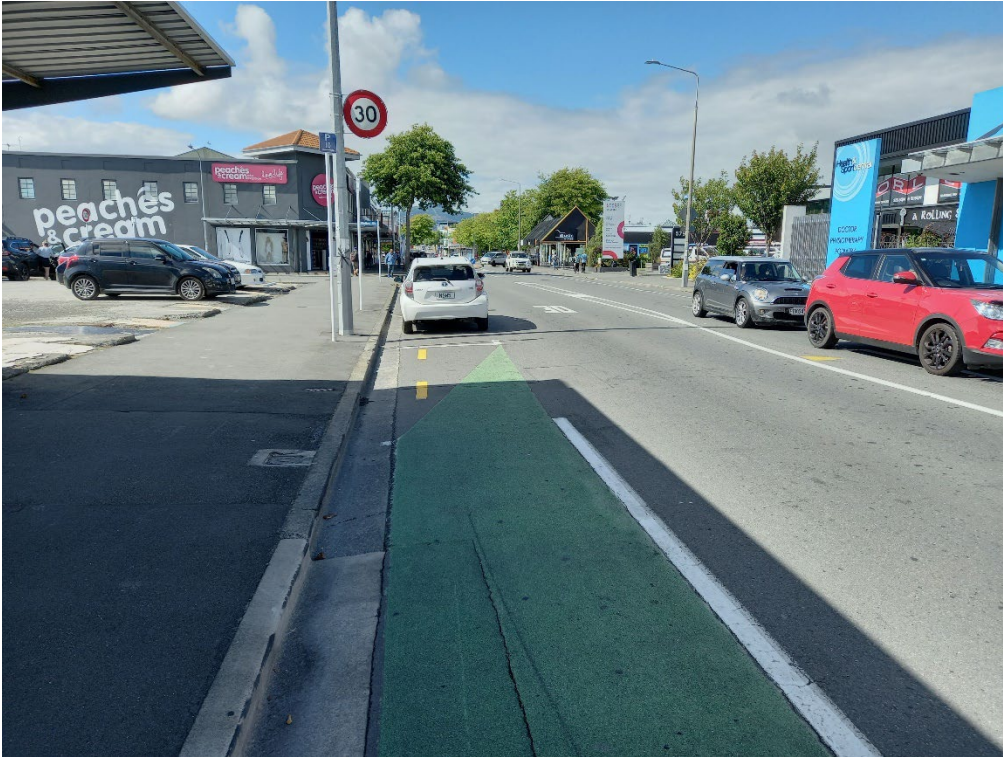
Figure 7.6 Cycle lane ends at parked car
