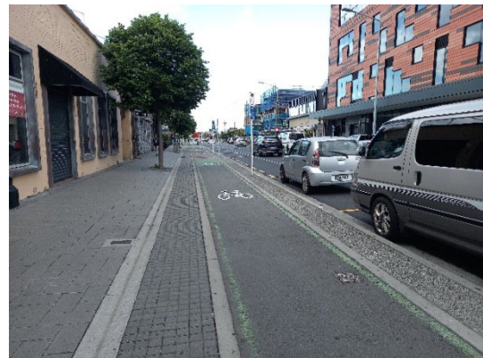
Figure 8.3: Separated cycleway next to parking
