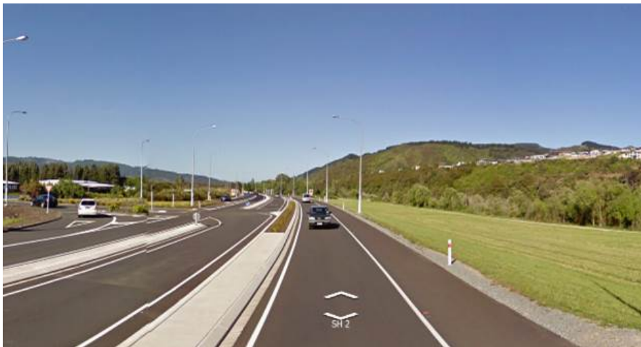
Figure 5.3 Seagull intersection with LTSL and give way sign, hit posts and painted seagull island
