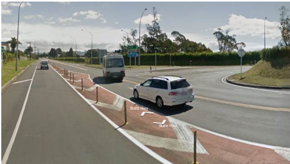
Figure 5.3 Seagull intersection with LTSL and give way sign, hit posts and painted seagull island
