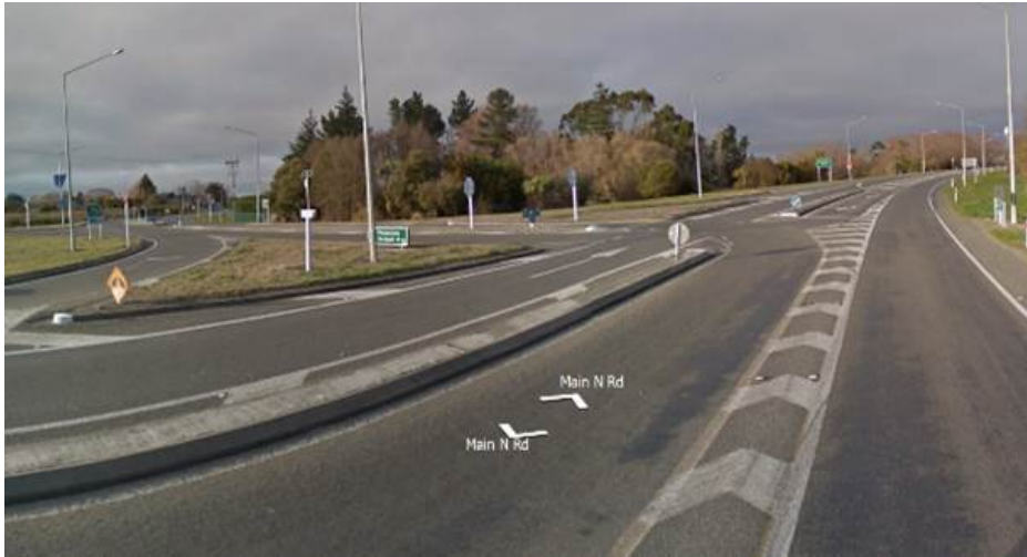
Figure 5.2 Seagull intersection with LTSL, solid seagull island and solid splitter island
