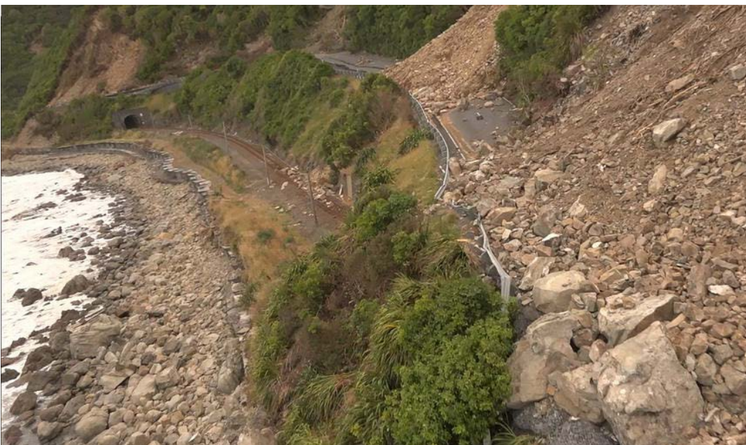
Figure 7.1 Damage to the road and rail network following the Kaikoura earthquake (Source: NZ Transport Agency)
