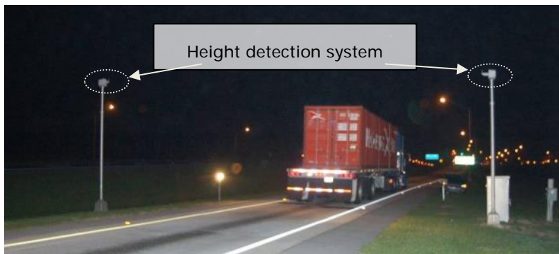
Figure 3.7 Example of a vehicle height detection system (Source: E- Squared Engineering)
