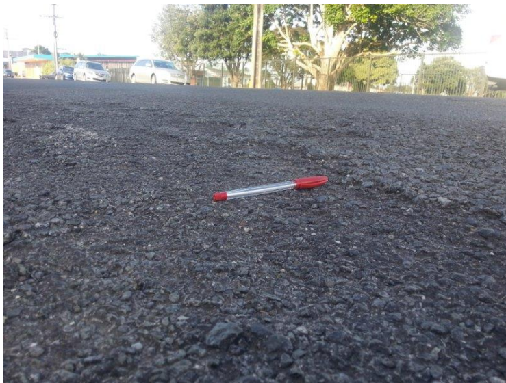
Figure 4.20 A closer view of the vertical height that exists when scabbing occurs in larger stone chipseals
