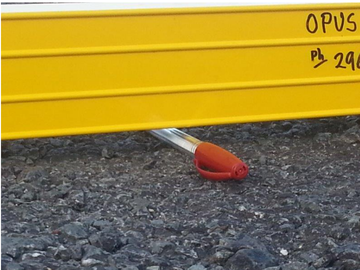
Figure 4.18 A closer view of a shallow depression that can be exaggerated when chip loss occurs at the same point. For larger size chip this depth can be greater than 5mm
