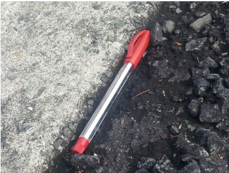
Figure 4.14 Scabbed surface or high lip at the channel often greater than 5mm
