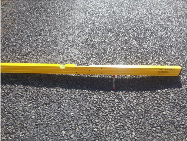
Figure 4.18 A closer view of a shallow depression that can be exaggerated when chip loss occurs at the same point. For larger size chip this depth can be greater than 5mm
