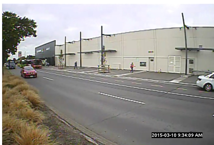
Figure 6.1 Site 1 Buckleys Road, Christchurch
