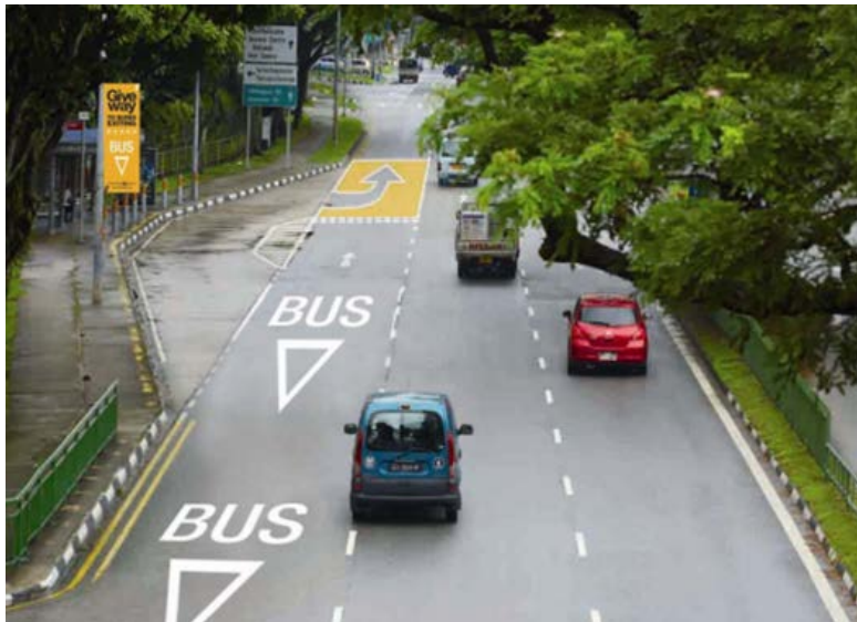
Figure 2.2 Singapore mandatory give way to buses road markings and bus bay (source: One Motoring 2014)
