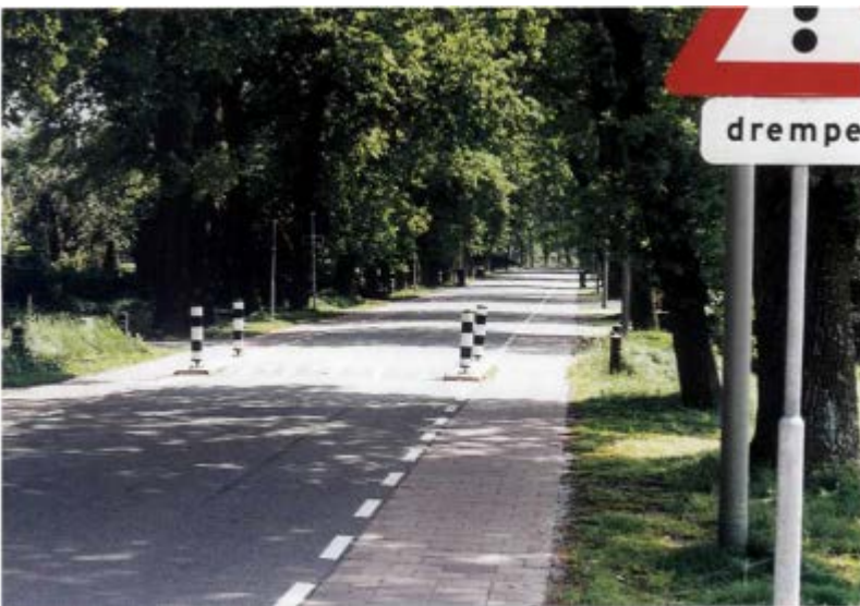
Figure 2.12 Designated bicycle lane edge strips paved with red brick on a Dutch rural access road, this time with bollards and speed cushion, and lines of evenly spaced trees at the road edge
