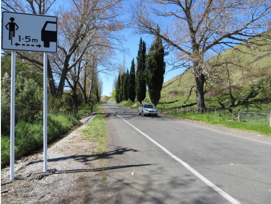
Figure 2.15 Tuki Tuki Road Hawke's Bay looking north, showing no centreline 2- 1 layout
