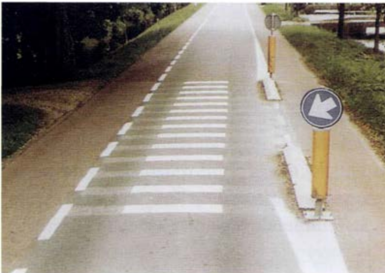
Figure 2.10 Broken longitudinal road markings and transverse lines, coupled with bollards and signage, to slow traffic on a Dutch low- volume, 60km/h rural road
