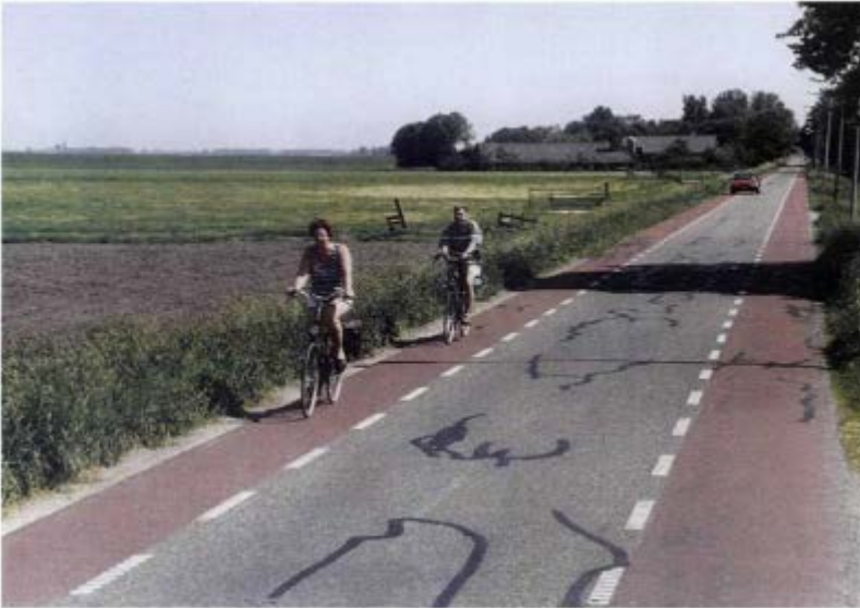
Figure 2.11 Designated bicycle lane edge strips being used by cyclists on a Dutch rural access road
