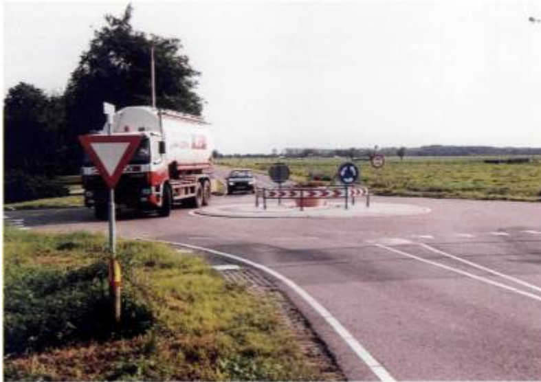
Figure 2.13 A roundabout at the junction of two 60km/h rural access roads in the Netherlands
