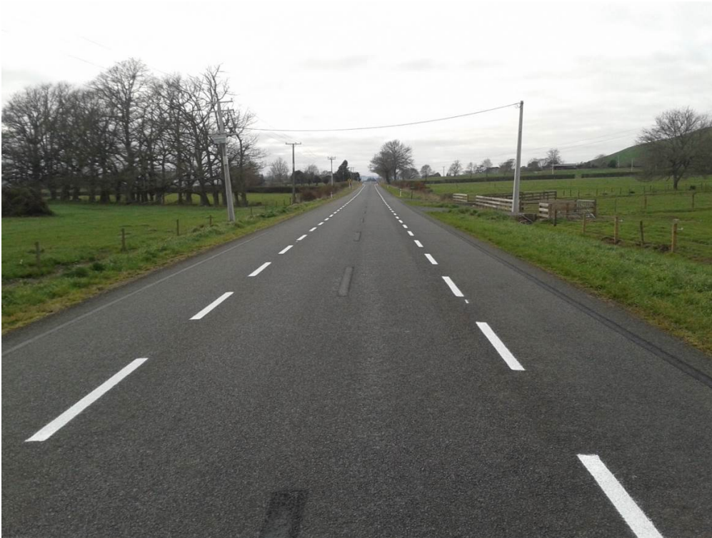
Figure 3.2 2-1 layout on Roto-o Rangī Road
