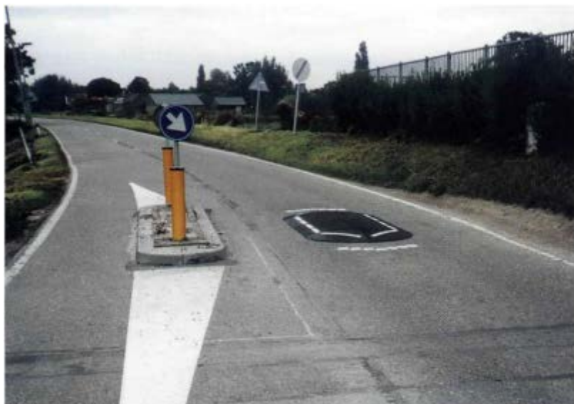
Figure 2.9 A traffic island, bollards and a speed cushion on a low- volume, 60km/h Dutch rural road
