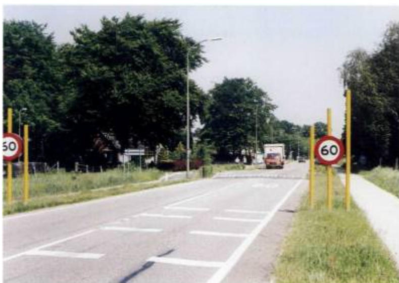
Figure 2.14 Measures used in the Netherlands to transition to a 60km/h rural access road, including bollard ‘gates’, posted speed limits, transverse road markings, roadway narrowing, and a speed bump
