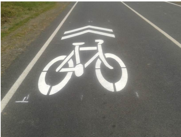
Figure 3.7 Sharrow markings used in on- road trial
