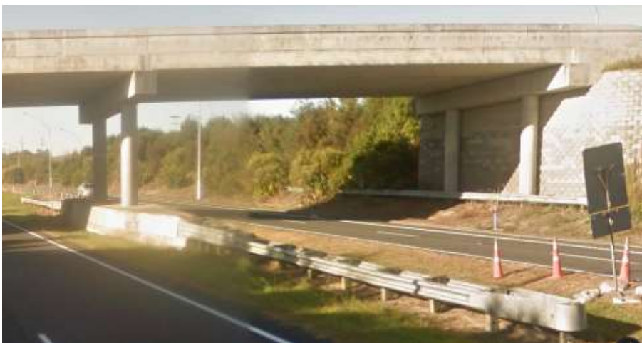
Figure 4.2 Example of short W-beam length
