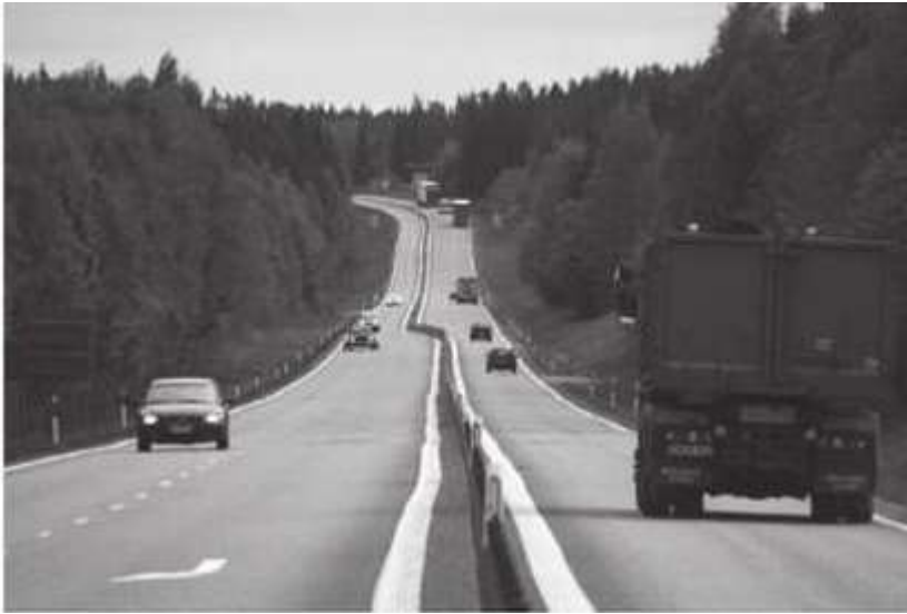
Figure 2.3 Example of 2 + 1 'collision free' roadway in Sweden
