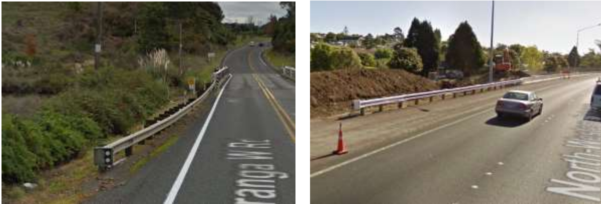
Figure 7.1 Examples of W-beam performing a capping function
