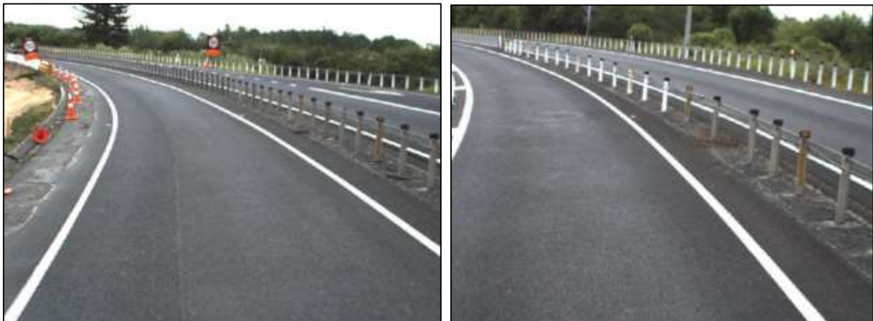
Figure 6.12 Median wire rope high incident site #1 SH01N RS 502 RP 434-900
