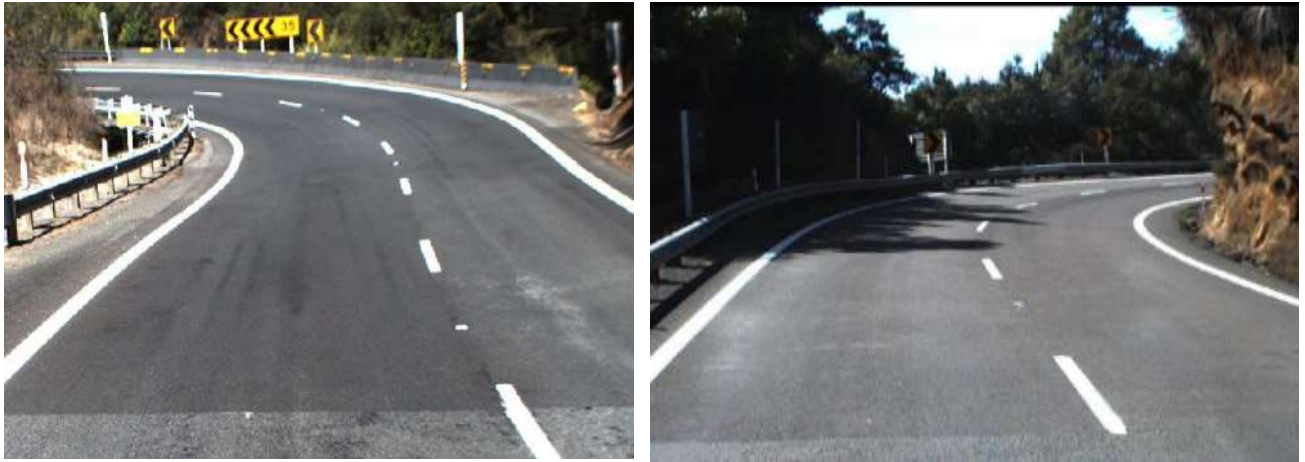
Figure 6.11 W-beam high incident site #3 SH01N RS 763 RP10000-11200
