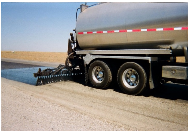
Figure 6.2 Spraying of PG76- 22TR (terminal blend)
