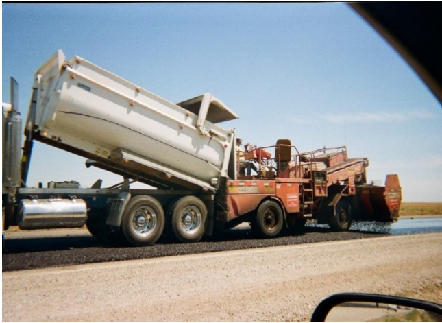
Figure 6.3 Application of hot chip in California
