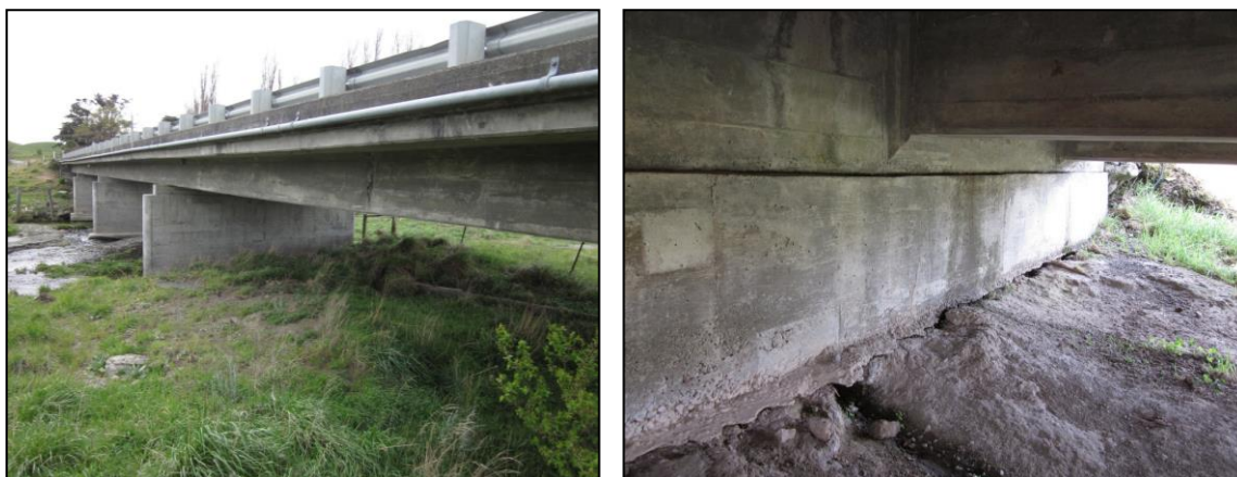
Figure 2.1 Flaxbourne River Bridge
