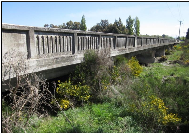
Figure 2.5 Hawkins River Bridge
