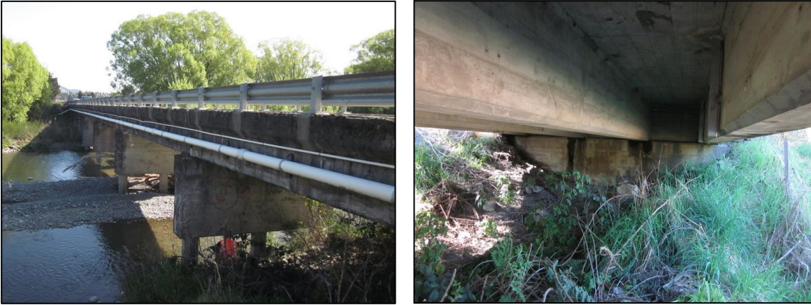
Figure 2.6 Selwyn River Bridge
