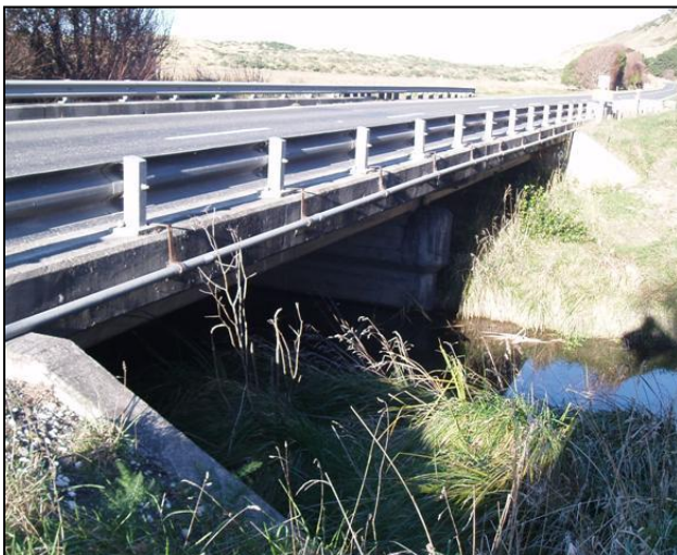
Figure 2.8 Tirohanga Stream Bridge
