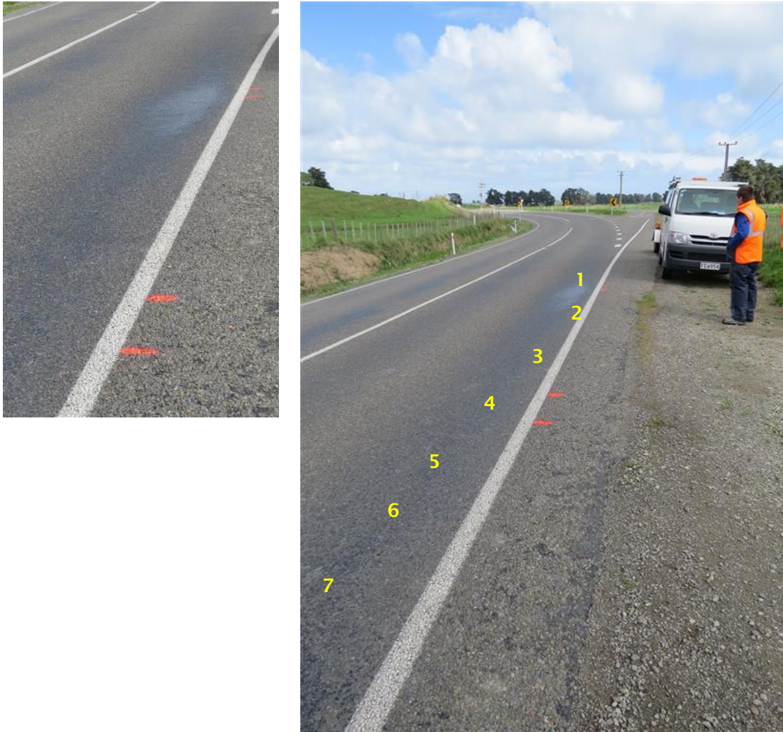
Figure 2.29 Site 1 showing flushed patch and core positions
