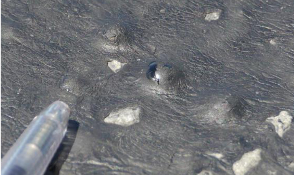
Figure 2.18 Bitumen blisters (SH77 Darfield)
