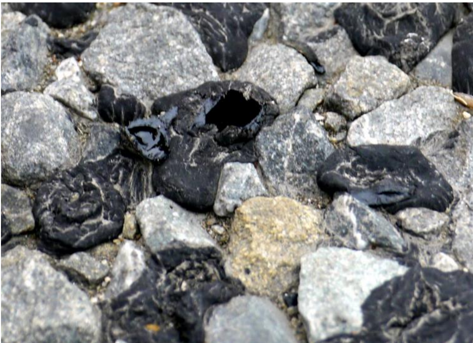
Figure 2.19 Blisters after cooling. The central blister has had the top removed to show the hollow interior (SH75 Banks Peninsular)
