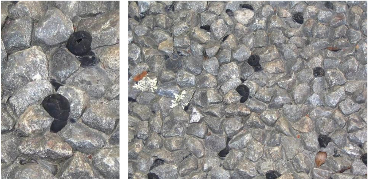
Figure 2.22 Bitumen blisters formed on an artificial seal constructed on a steel plate and exposed outdoors
