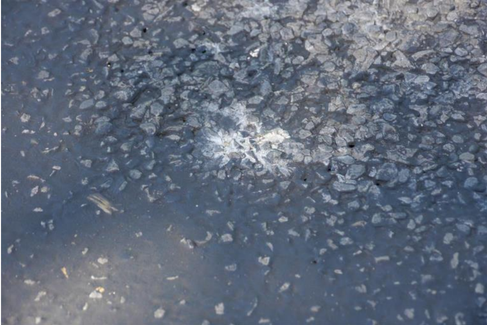
Figure 2.60 Site 6, vent holes and basecourse fines in flushed patch
