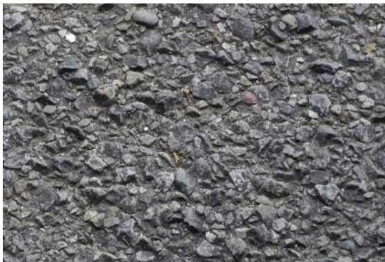
a) Two-coat seal
