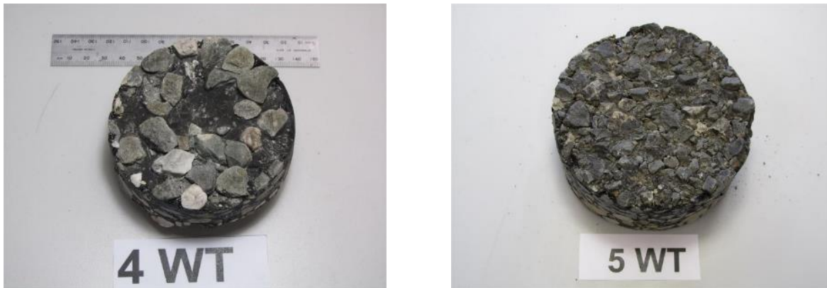
Figure 2.16 Wheel track cores from SH8 (left) and SH5 (right), sites used to verify the OMD test, note the chip loss from the SH8 core
