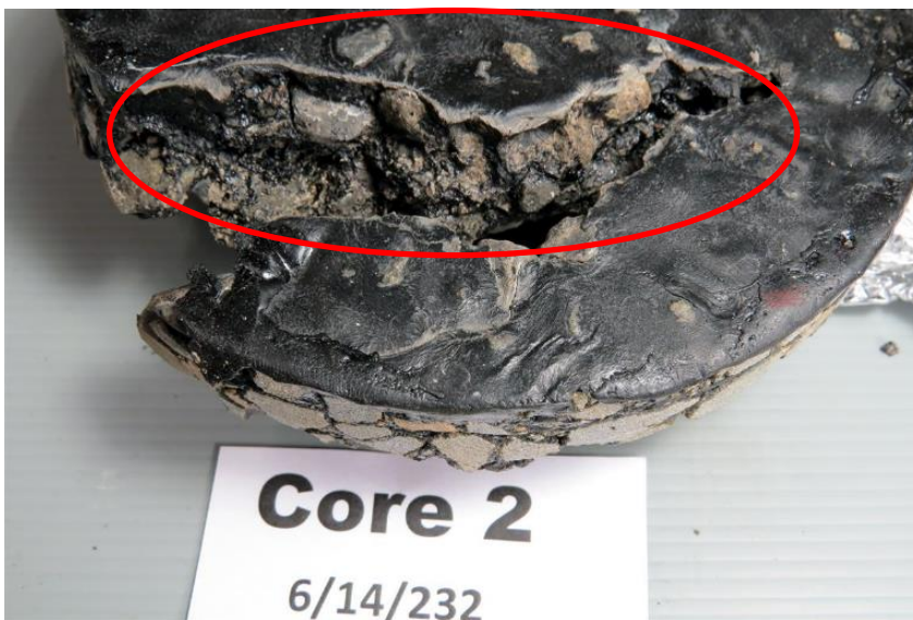
Figure 2.34 Site 1, crack in core 2 opened to reveal stripped clean aggregate on the sides of the crack
