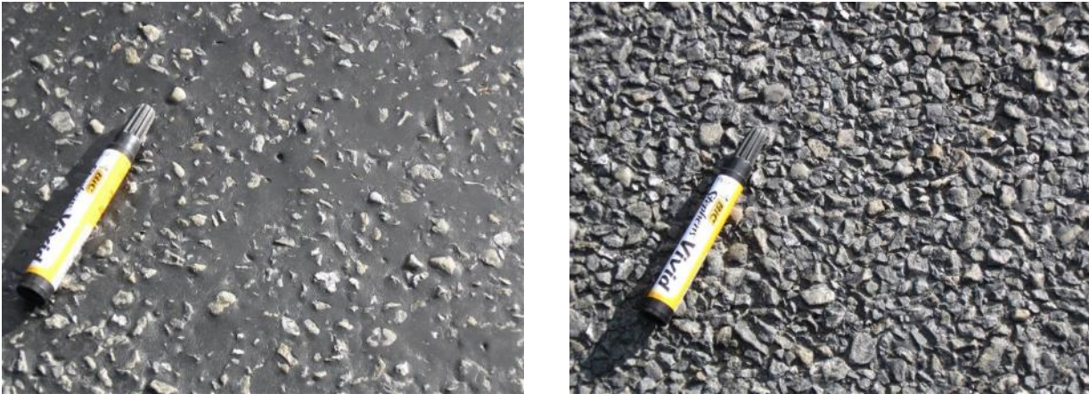
Figure 2.64 Site 7, flushed patch texture showing venting holes and adjacent well- textured seal
