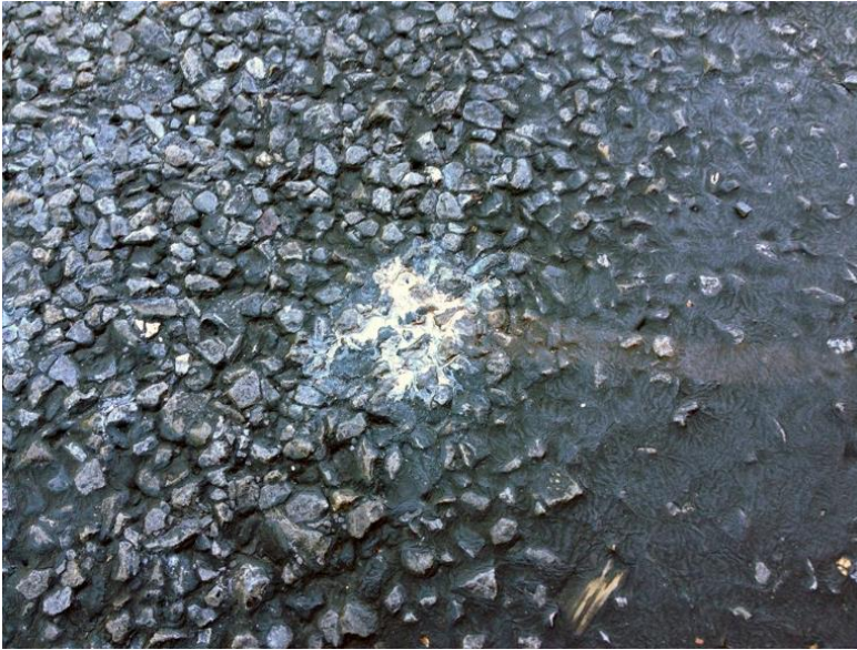
Figure 2.55 Site 5, specimens from textured area and partially flushed seal showing the full depth of the seal layer down to the (bitumen bound) basecourse. An asphalt layer is present two seal coats down from the surface. Stripping in this layer core 8 resulted in failure when extracting the core
