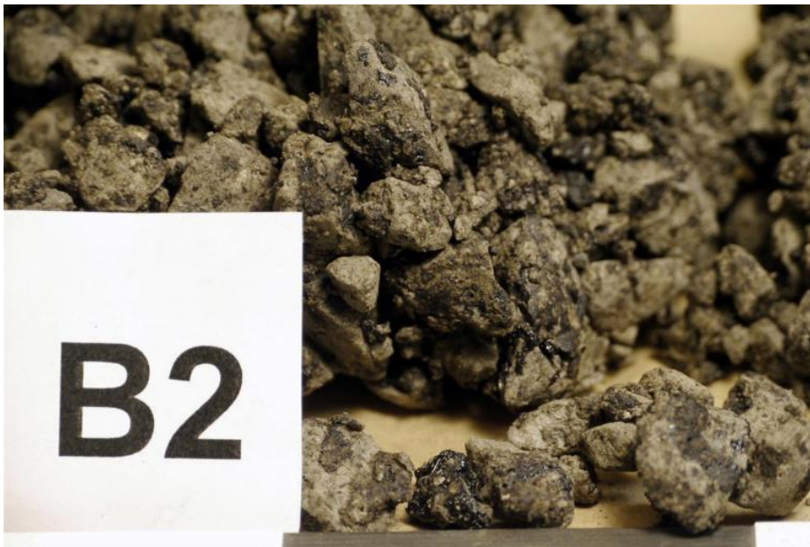
Figure 2.52 Site 4, material from the bottom of flushed patch specimen showing stripped aggregate
