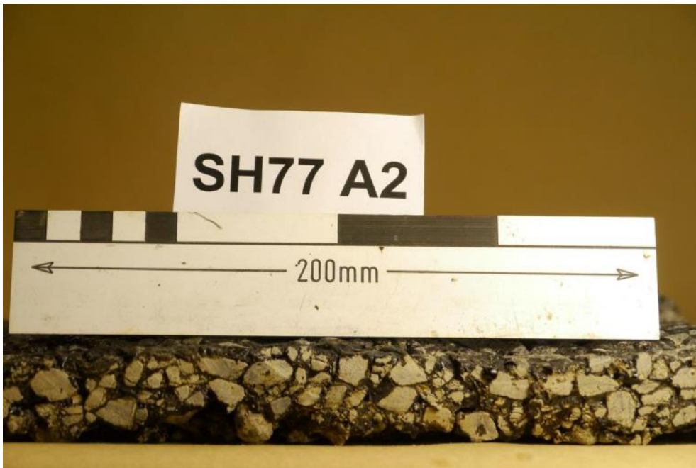
Figure 2.44 Site 3, profile of specimen from a flushed area
