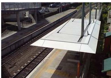
Kingsland station has been upgraded in stages from 2004 when it was rebuilt for western line double-tracking, 2006 platform lengthening and 2011 when shelters were built for the rugby world cup. (WP)
