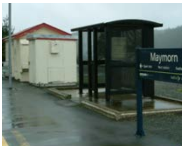
Maymorn (left-hand photo) is on the Upper Hutt side of the Rimutaka hill range and has had a new 'bus stop' style shelter installed..
