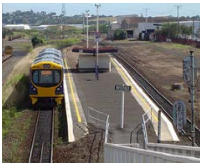
Pukekohe station which has not been refurbished and features ramp access (WP)
