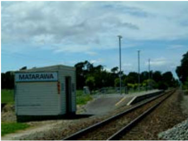
Matarawa station is between Greytown and Carterton and has a very sparse catchment. The platform has been upgraded with a new ramp and lighting.
