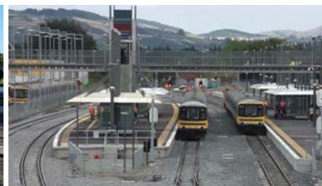
The platforms at Papakura were lengthened in 2007 and the station rebuilt in 2012/13 on the western side of platform with a refurbished ticket office.
