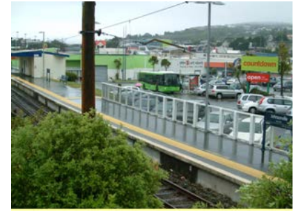
Johnsonville is the terminal station at the end of the 11km rail line. It is the busiest station and was being repainted when it was photographed in December 2014. There is car parking and the Johnsonville hub for Mana Coaches. (NJD)
