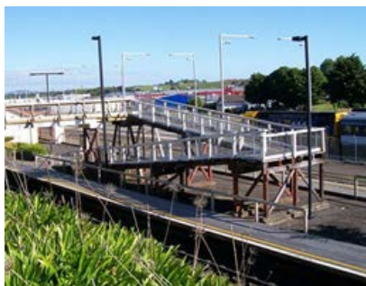
Westfield station has a walkway to an overbridge. The station had not been upgraded at the time of the survey as the station's future has been under review. (WP)
