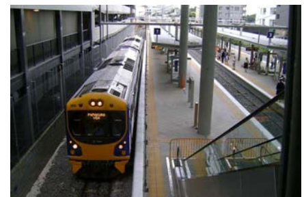
Newmarket station, upgraded in 2010 with four platforms and escalator/lift platform egress via an overhead walkway is the second 'hub' station on the Auckland rail network (WP)
