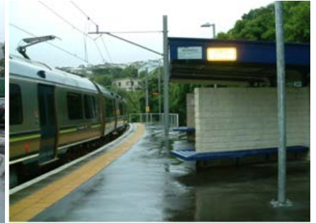
Like all the Johnsonville line stations, Awarua St has had its platform raised and resurfaced to accommodate the new Matangi trains. Electronic train indicator boards. (NJD)
