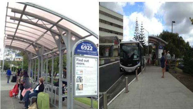
Two photos of the bus stop at near Westfield train station and shopping mall. The stop has shelter, seating, electronic and standard timetable information and is in a very good condition. (CH)
