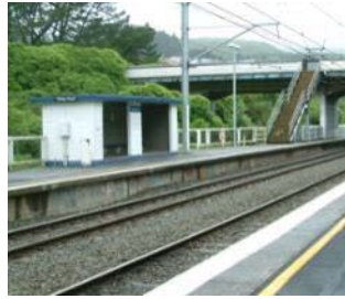
Takapu Road has stair access from the main road and a ramp access from a minor road. (NJD)
