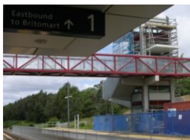
New overbridge with lifts being constructed at Swanson station. (AKTNZ)
