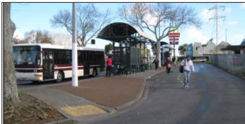
Figure 5.14 Otara bus interchange prior to upgrade
