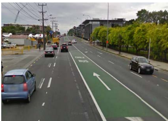
Median bus lane – Wairau Road, Auckland
