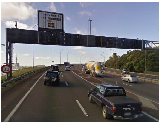
Auckland Harbour Bridge (Northern Motorway), Auckland. Moveable barrier allows kerbside lane to be reserved for buses
