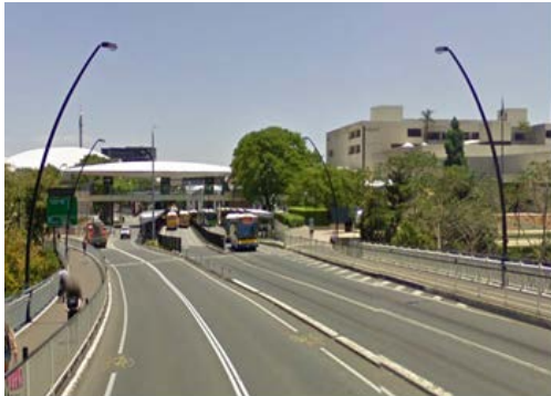
Victoria Bridge (South East Busway), Brisbane, Australia
