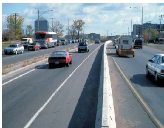
I-394 Minneapolis (temporary arterial HOV lane)
