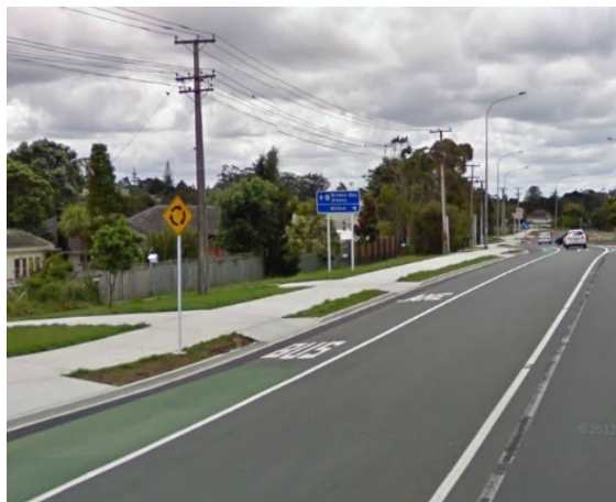
East Coast Road, Auckland (approach to a roundabout)
