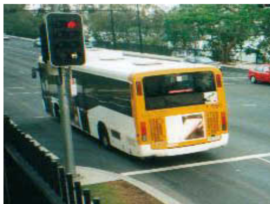
Coronation Drive, Brisbane (now removed). Central reversible lane allows kerbside lane to be reserved as a bus lane in peak periods
