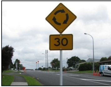
Figure 2.9 Roundabout sign with 30km/hr advisory speed sign, installed on approaches to the C-roundabout
