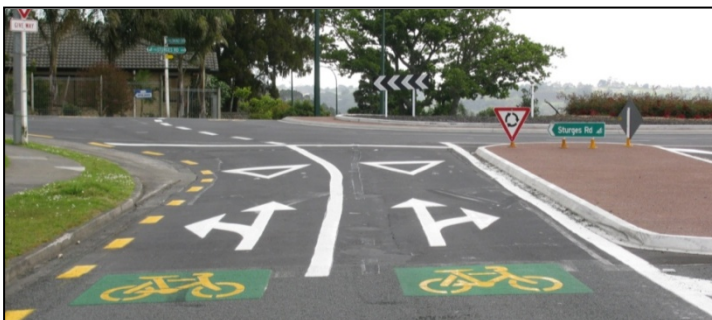
Figure 2.41 Cycle symbol road markings installed on northern and southern approaches to the Palomino Dr/Sturges Rd C-roundabout 5
