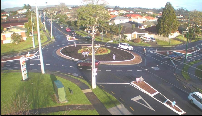
Figure 2.7 Palomino Dr/Sturges Rd C-roundabout, north approach with truck lane-use sign and cycle symbol road marking 3
