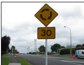
Figure 2.12 Roundabout sign with 30km/hr advisory speed sign, installed on approaches to the C-roundabout
