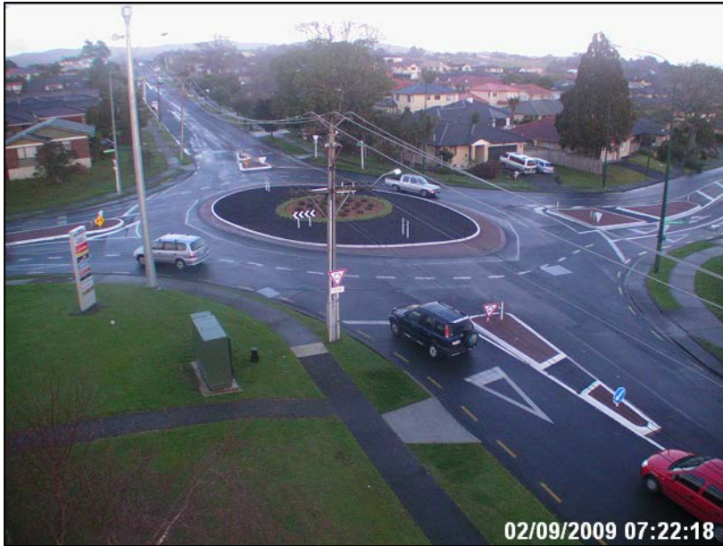
Figure A.1 Camera view for video survey done after Palomino Dr/Sturges Rd roundabout was converted to a C-roundabout
