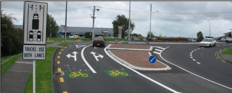
Figure 2.8 Palomino Dr/Sturges Rd C-roundabout, cycle symbol road marking on circulating lanes in roundabout
