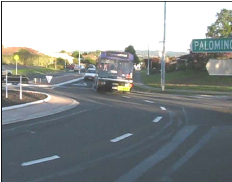
Figure 2.14 Photo of incorrect lane use by a bus on the Palomino Dr approach to Palomino Dr/Sturges Rd roundabout
