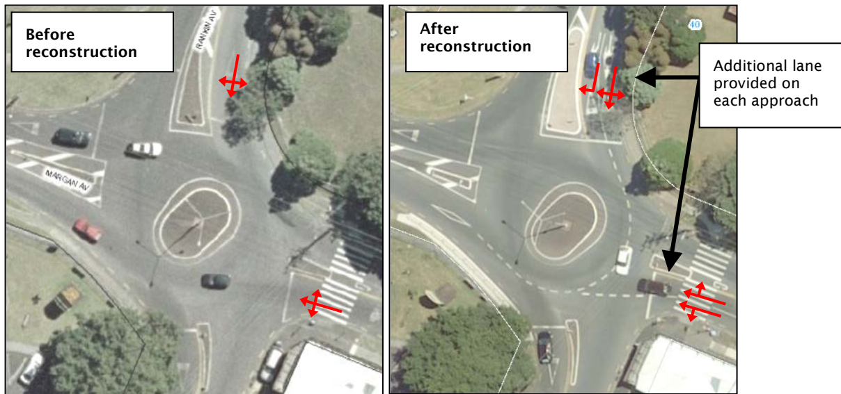
Figure 3.7 Aerial photos for the Margan Ave/Hutchinson Ave roundabout prior to and following reconstruction in November 2007
