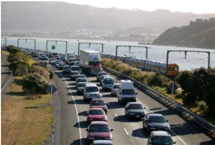
Figure 5.3 Wellington SH1 road and rail corridor Porirua Harbour
