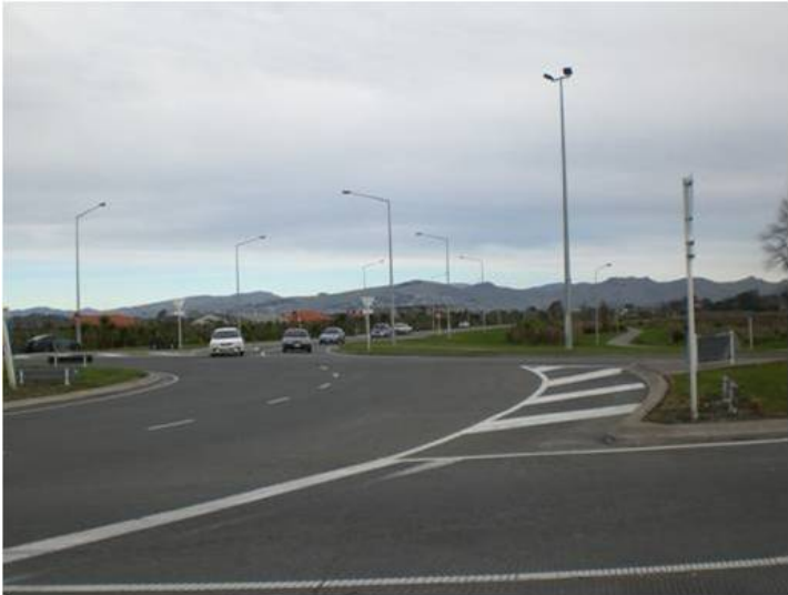
Figure F.17c Queen Elizabeth II and Anzac Drive Bridge and roundabout
