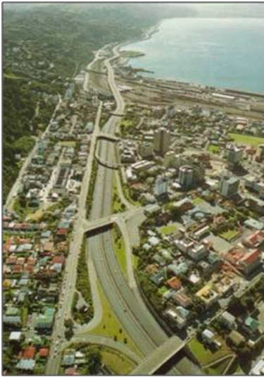
Figure 5.1 Wellington waterfront motorway (looking north)
