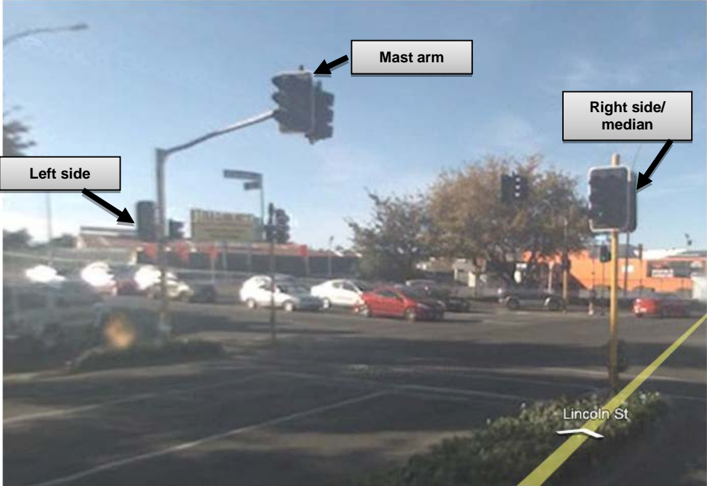
Figure 4.5 Location of signal displays on left side of approach, median and mast arm (Google Street View image)
