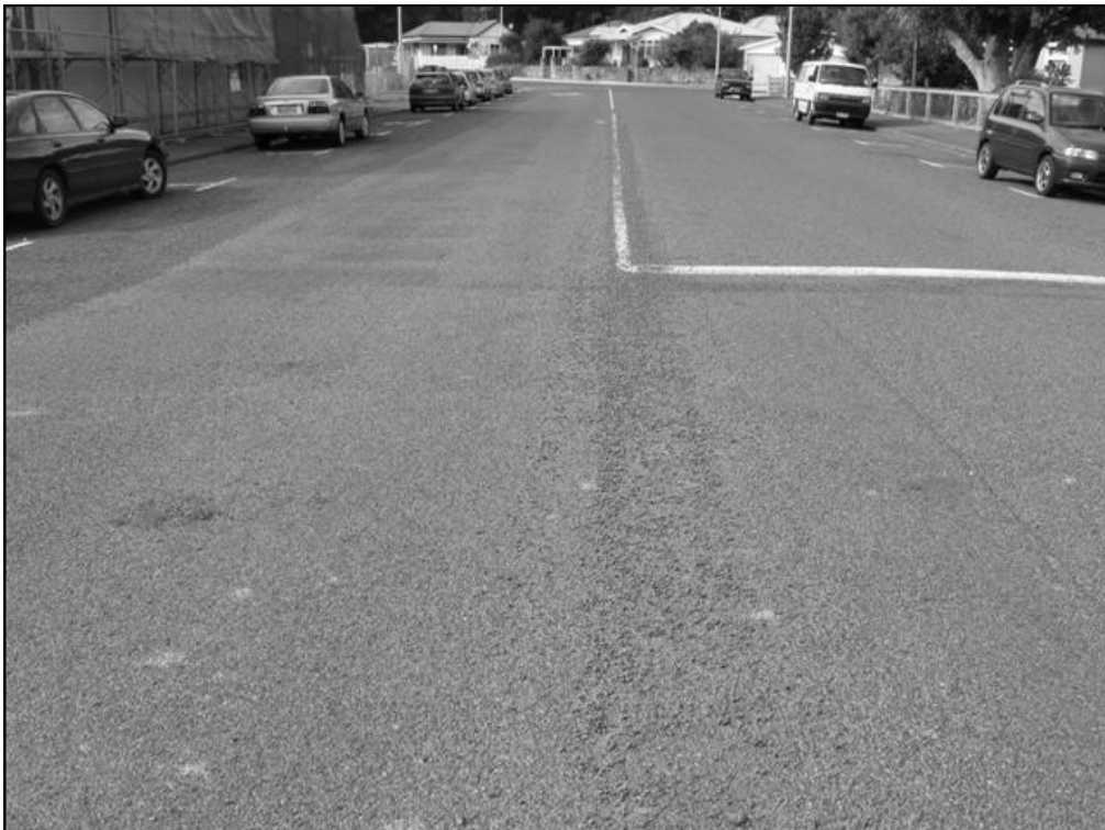
Figure 6.8 August 2009: chip loss on centre line
