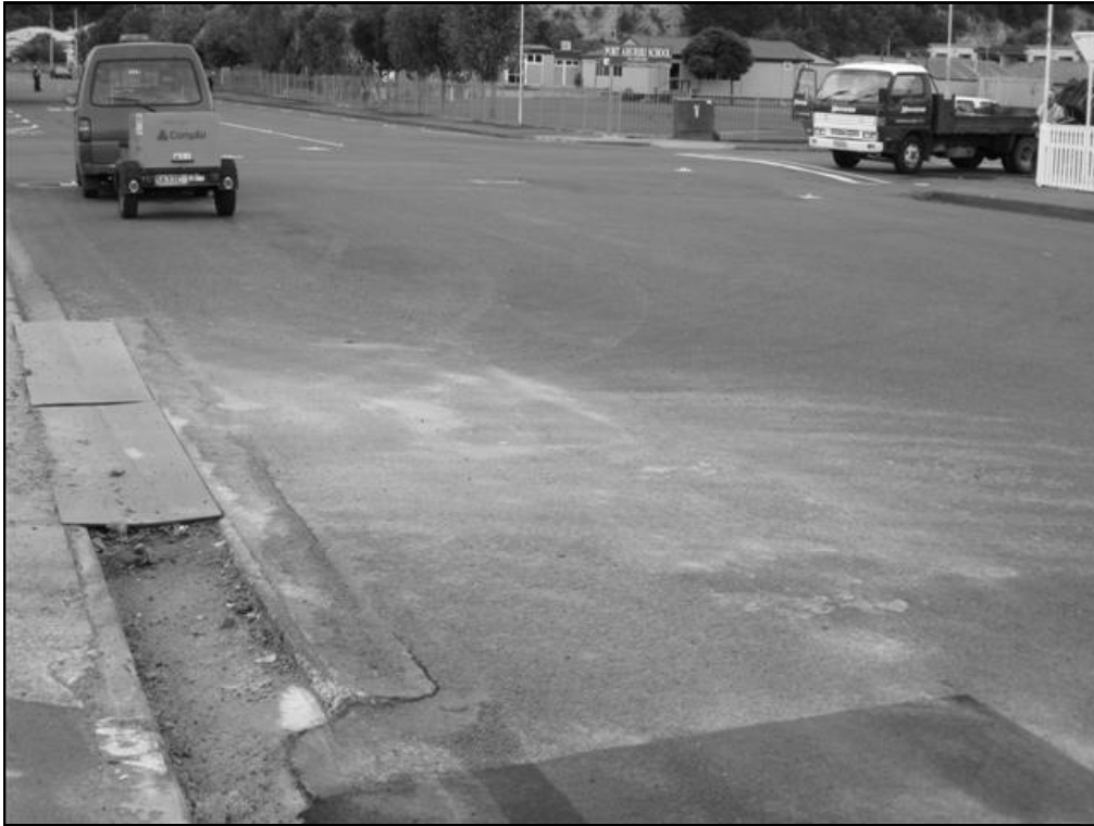
Figure 6.2 13 March 2009: Lever Street-Domett Street intersection before sealing
