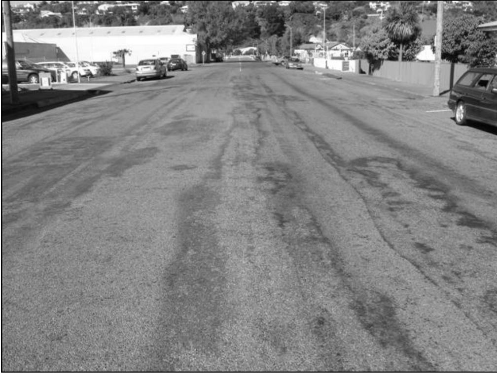
Figure 6.11 April 2011: looking towards Domett Street, showing flushing of the repairs
