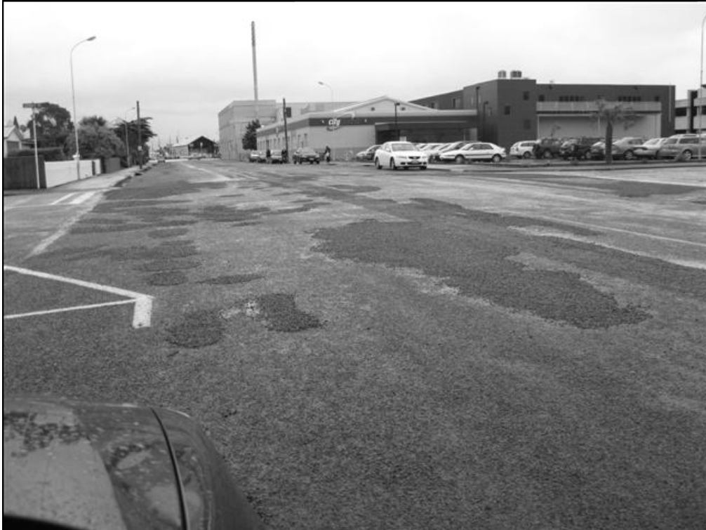
Figure 6.10 July 2010: repairs at the Lever Street-Domett Street intersection
