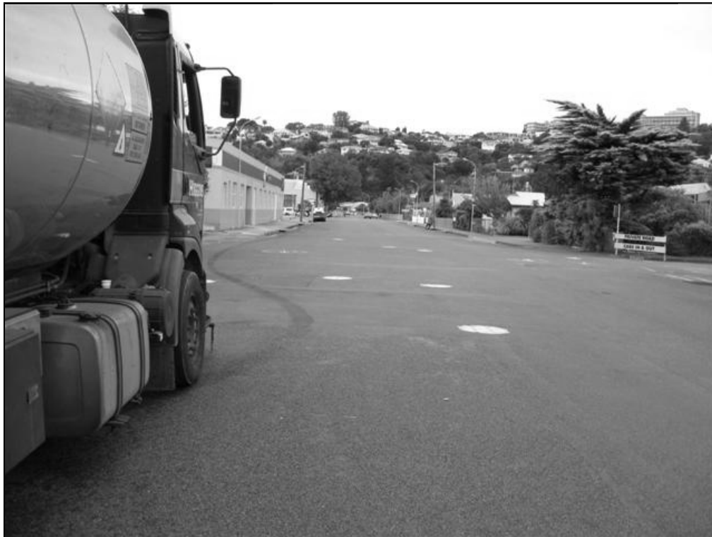
Figure 6.1 13 March 2009: Lever Street before sealing
