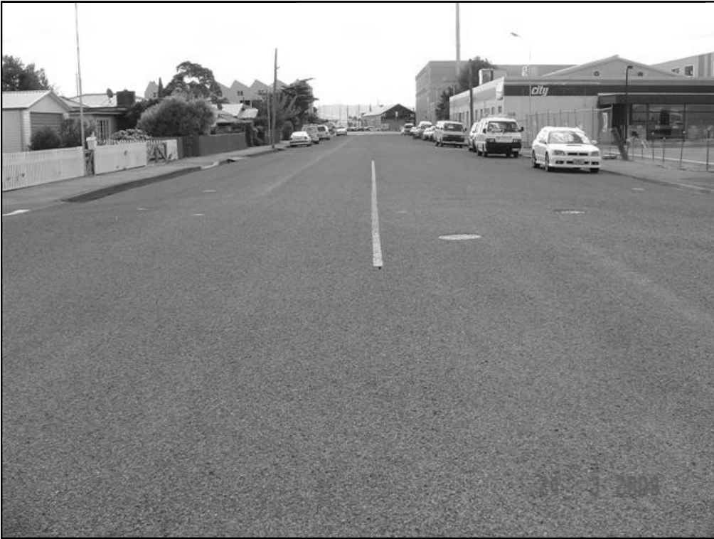
Figure 6.6 24 March 2009: alternative view of completed seal
