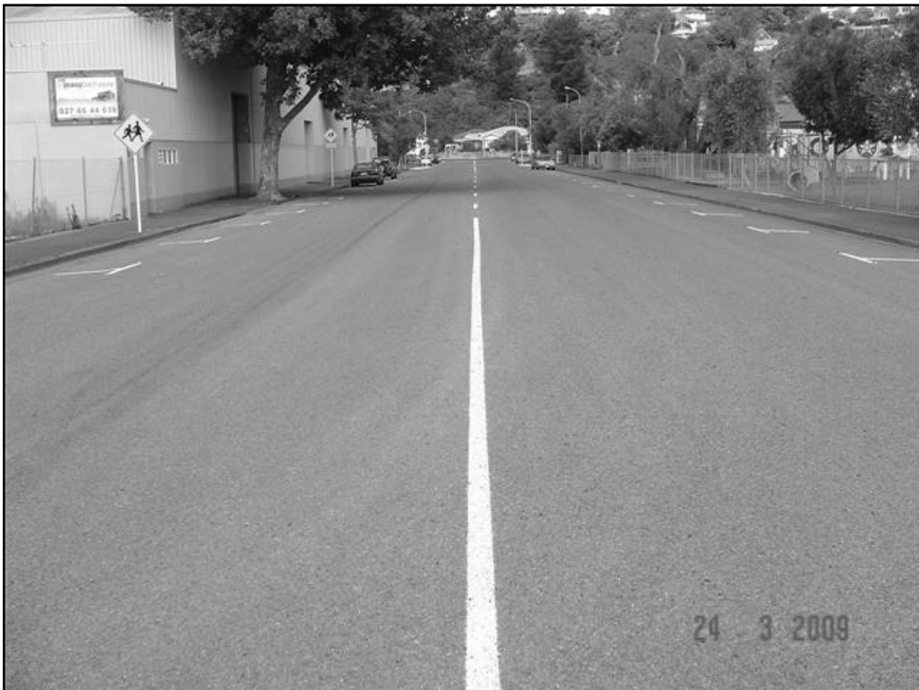
Figure 6.5 24 March 2009: completed seal on Lever Street
