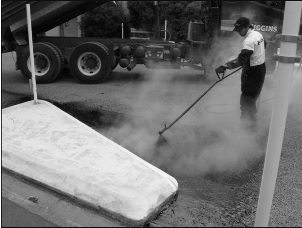
Figure 6.4 The hand lancing stage of applying the test seal
