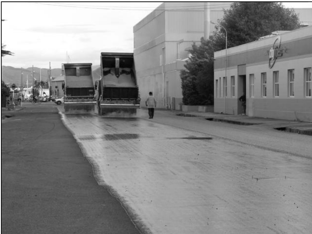
Figure 6.3 Applying chip to the Lever Street test site
