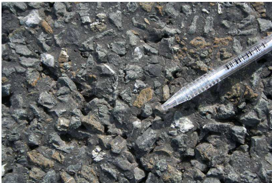
Figure 4.1 Retextured OGPA surface (note the newly formed faces)
