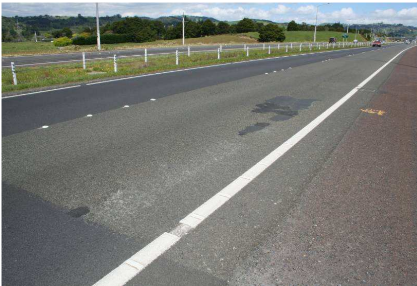
Figure 4.7 Pavement rutting and subsequent failure of the OGPA surfacing
