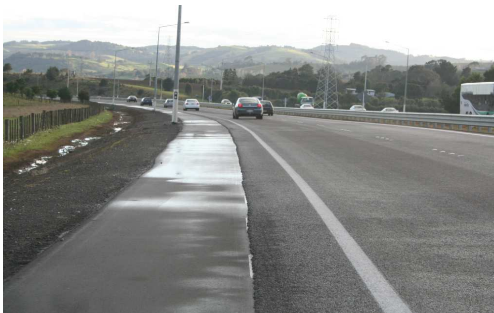
Figure 4.4 Free-draining OGPA on the South Auckland Motorway
