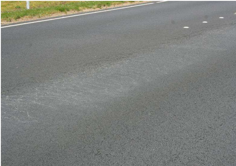
Figure 4.7 Pavement rutting and subsequent failure of the OGPA surfacing
