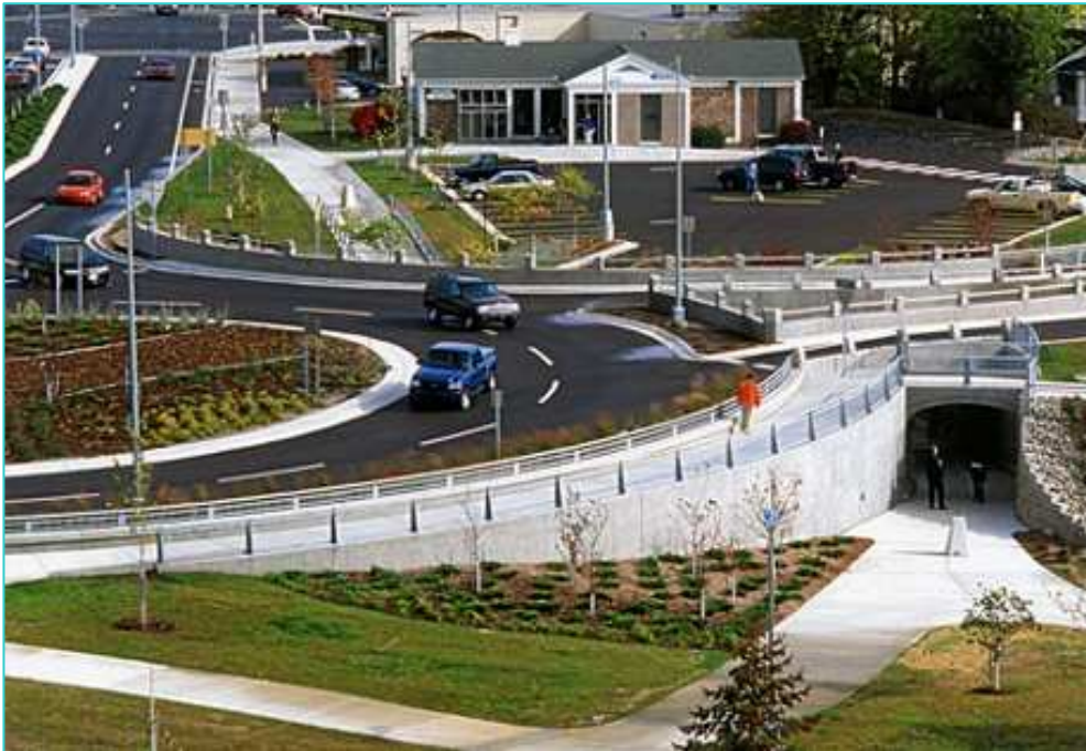
Figure 3.31 Underpass for cyclists, US (image inverted) (unknown source)
