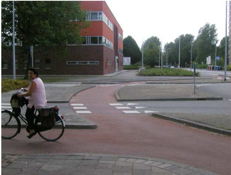
Figure 3.30 Cyclists' path around a roundabout that does not allow cyclist priority (Christchurch City Council)
