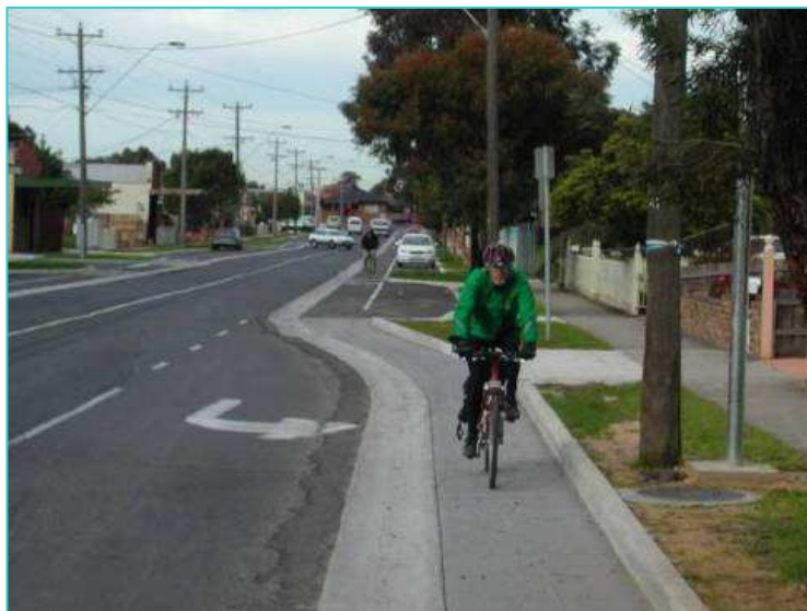
Figure 3.11 Kerbed cycle lane with parking (in background of picture), Melbourne, Australia (H Barber)
