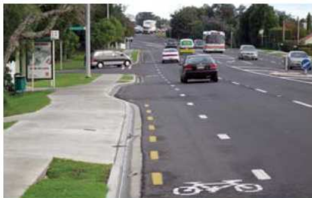
Figure 3.8 Kerbside cycle lane, North Shore City, New Zealand (LTNZ 2005, p36)
