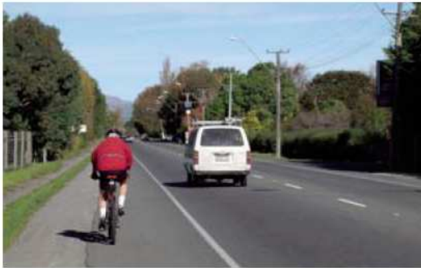
Figure 3.2 A wide sealed shoulder on Marshland Rd, Christchurch, New Zealand (LTNZ 2005, p38)
