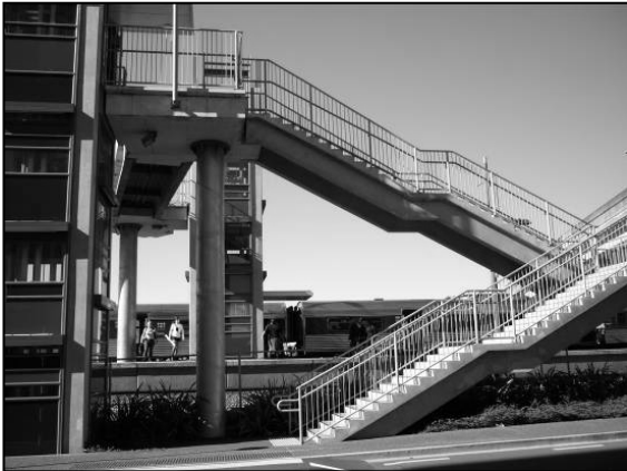
Figure 1.3 Pedestrian facilities (ramps and lifts) linking the train station to the main Sylvia Park complex
