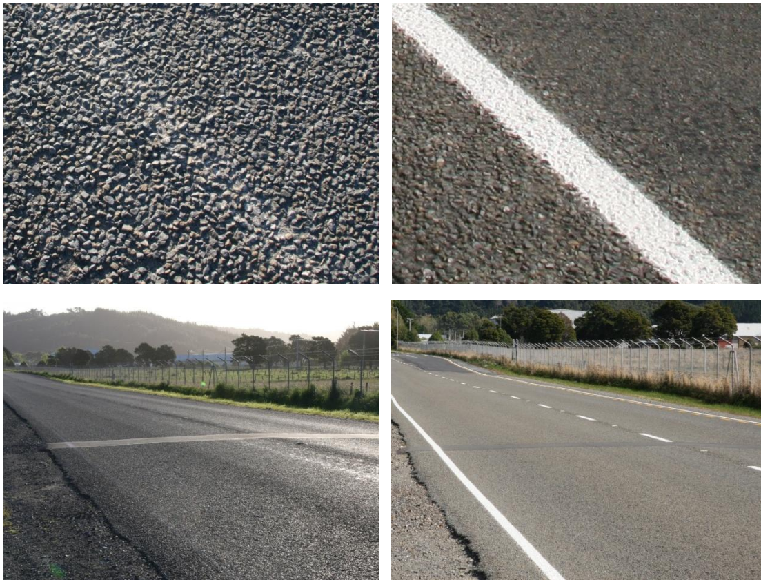
Figure 3.2 Linemarkings before (left) and after (right) an upgrade
