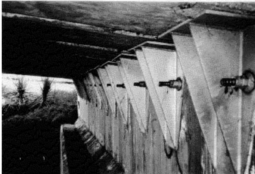
Figure 5.7 Seismic strengthening of a bridge deck to abutment connection.
