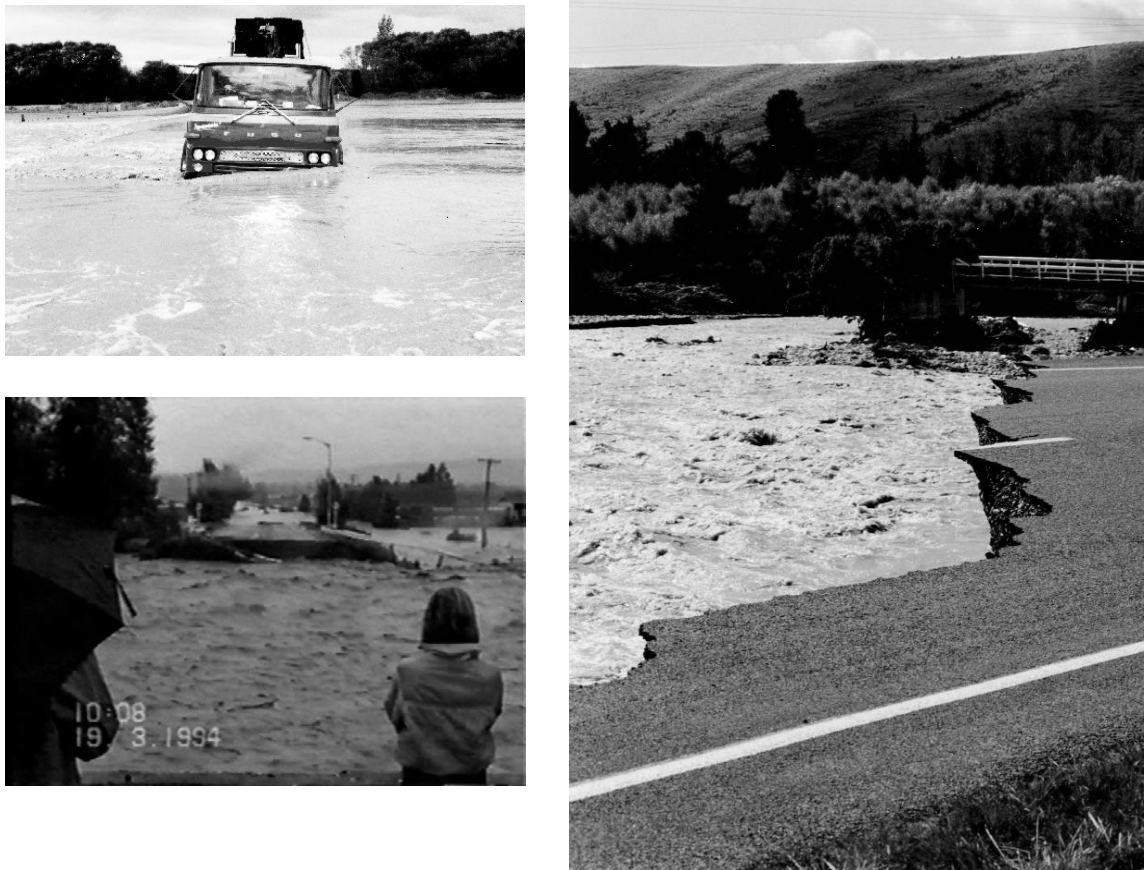
Figure 8.2 Effects of flood hazard can include significant disruption of road networks.
