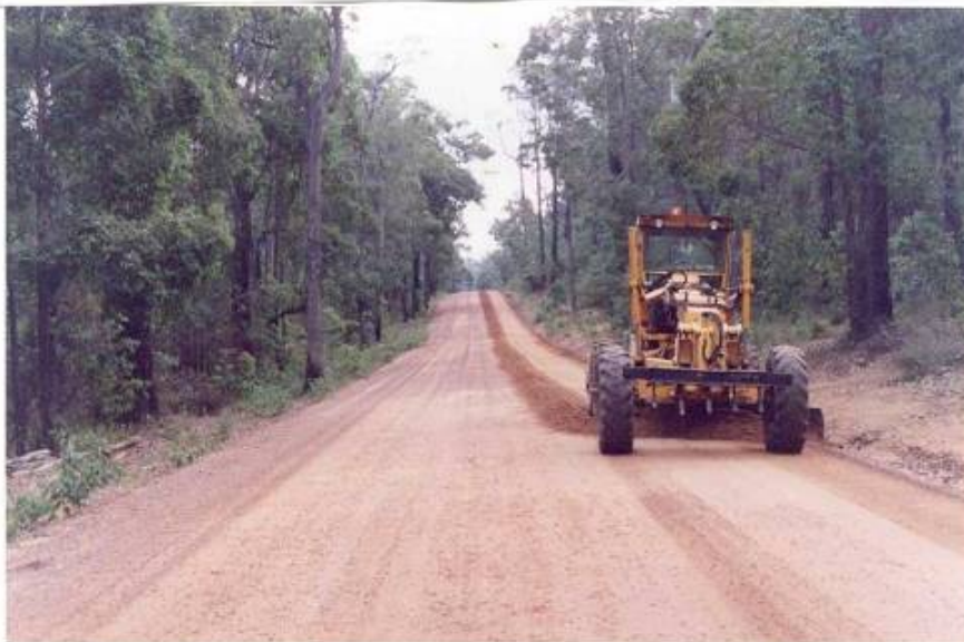
Figure 5.1 Periodic maintenance practice.
