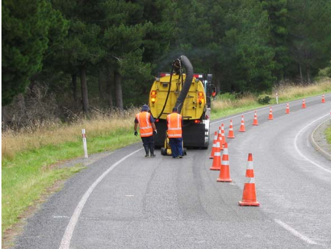
Figure 4.13 Watercutting on Wishing Well site facing southwest.
