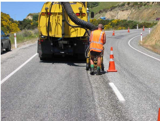
Figure 4.3 Watercutting at Tunnel Hill.
