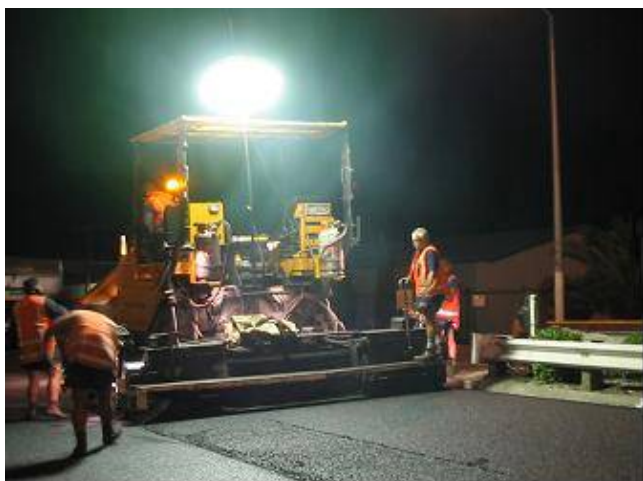
Figure 4.16 Laying SMA on Rosebank site.
