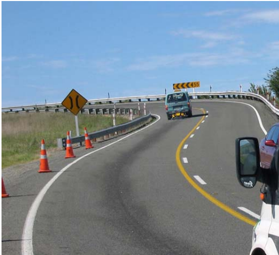
Figure 4.5 Griptesting between the wheelpaths at Tumai Overbridge site.
