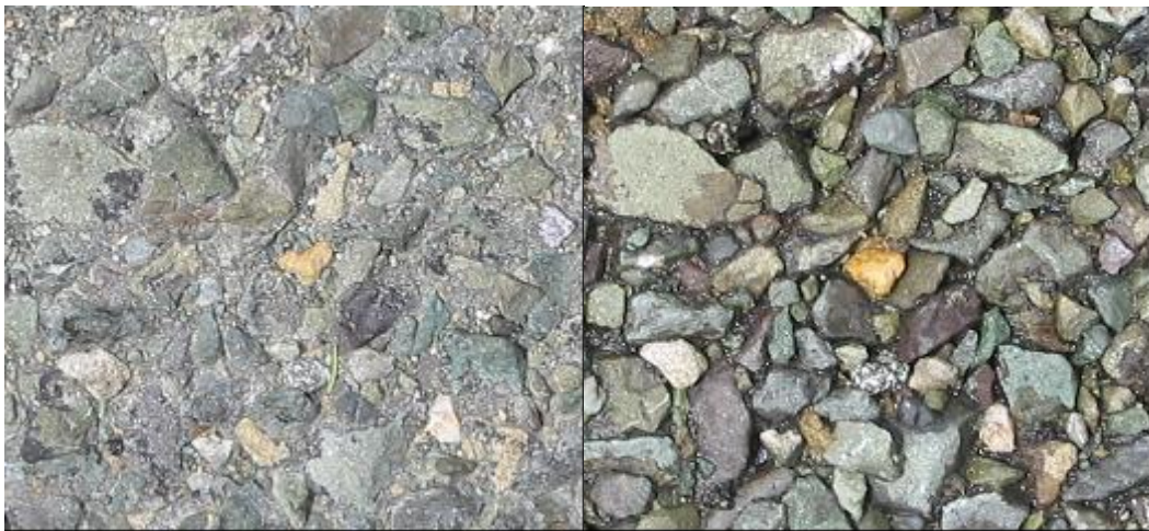
Figure A1. Whangamoia Saddle – surface before and after watercutting.
