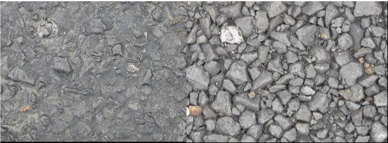
Figure A4 Poppellwells Surface before (left) and after (right) watercutting.
