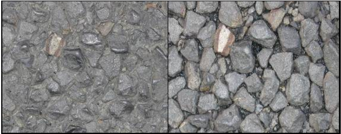
Figure A3 Wishing Well before (left) and after (right) watercutting.
