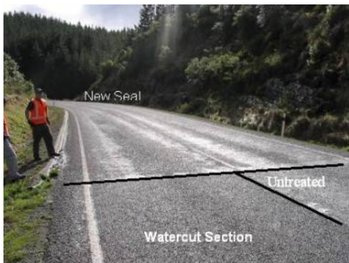
Figure 6.4 New chipseal on Wishing Well site six months after construction.
