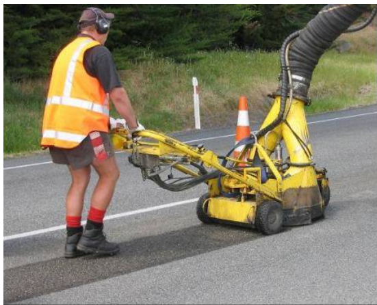
Figure 3.1 Watercutting during the Tai Tapu trials.
