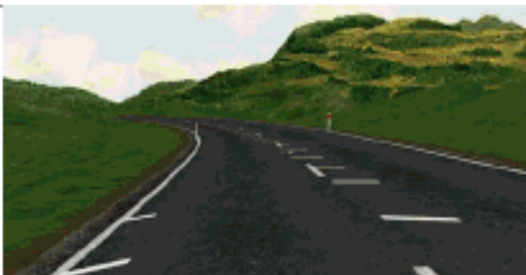
7: PW 17 & herringbone markings. Effectiveness rating (1 to 7) _____ Practical utility rating (1 to 7) _____
