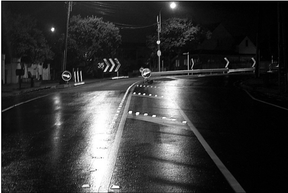
Figure J2: Night view of a pedestrian refuge island with a 'no overtaking' line and rrpms on approaches.
