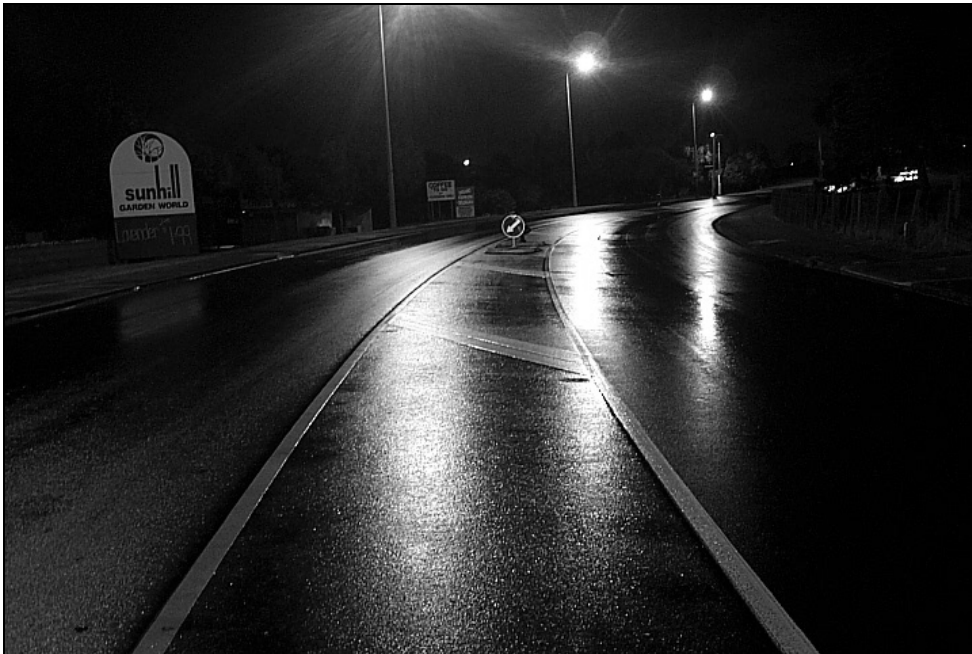
Figure J1: Night view of a pedestrian refuge island with standard markings.
