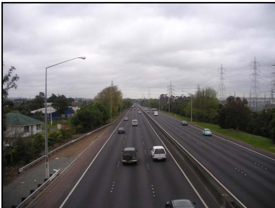
Figure 7.2 Northbound lanes on Location 1 on the Southern Motorway, Auckland.
