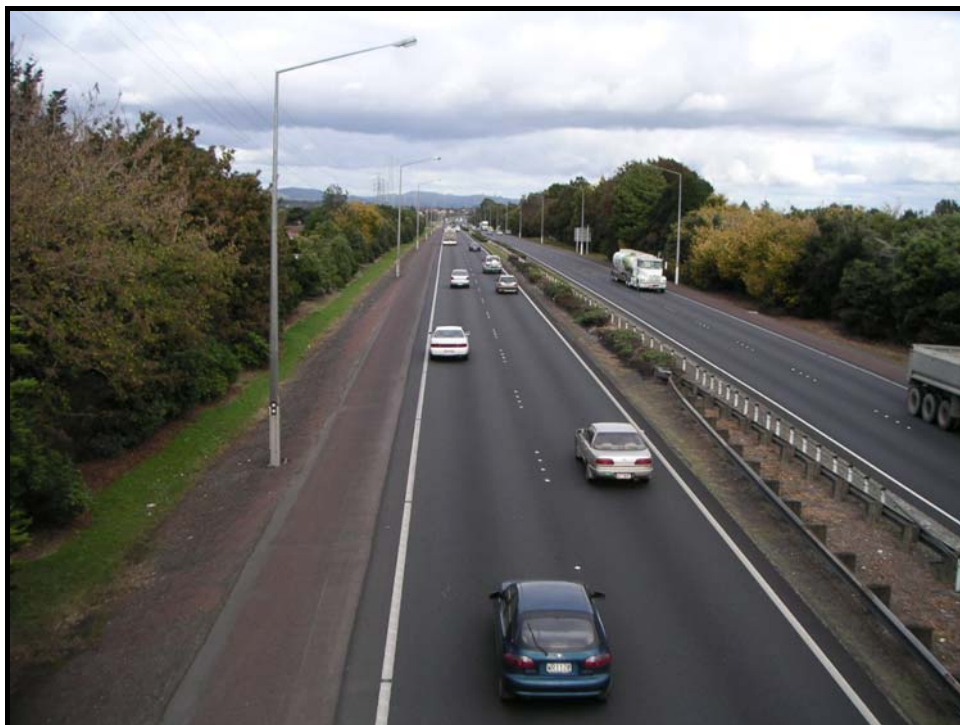
Figure 7.6 Southbound lanes at Location 2 on Southern Motorway, Auckland.
