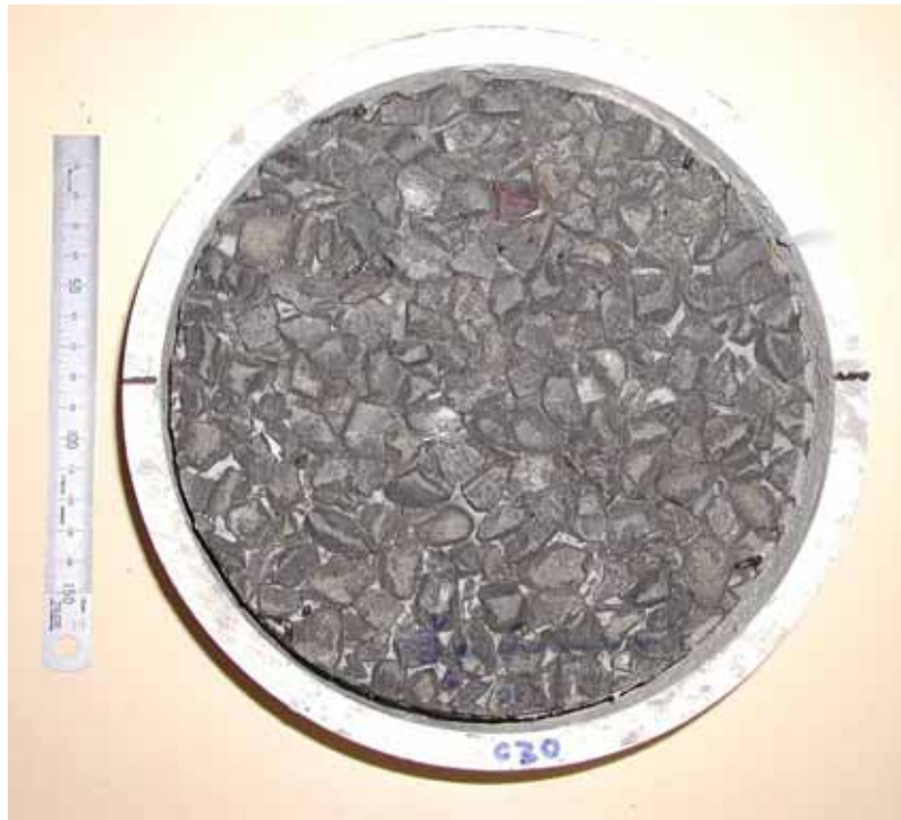
Figure A4.3 Pound Road aggregate, grade 3, left wheelpath, 'high' HCV passes (direction of traffic = ↔).
