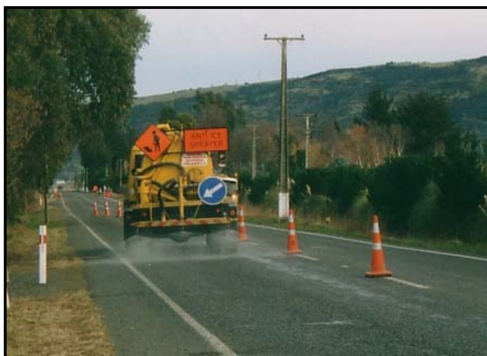
Figure 2.1 Applying CMA in liquid form on a Coastal Otago state highway.
