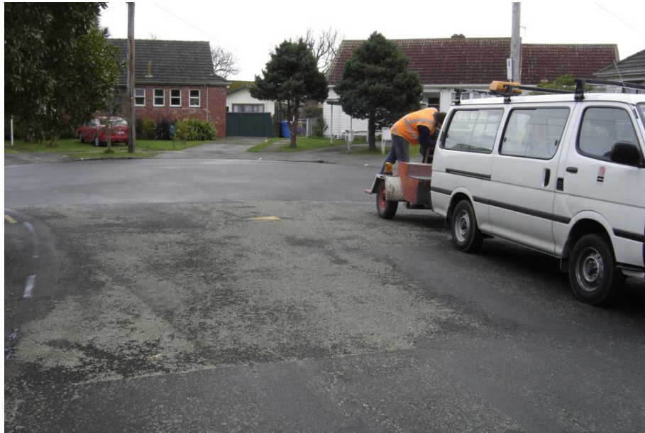
Figure 2.1 View of typical grade 3 seal surface (with lichen).
