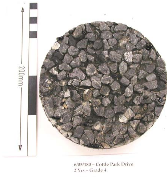
Figure 2.3 Core before bitumen extraction.
