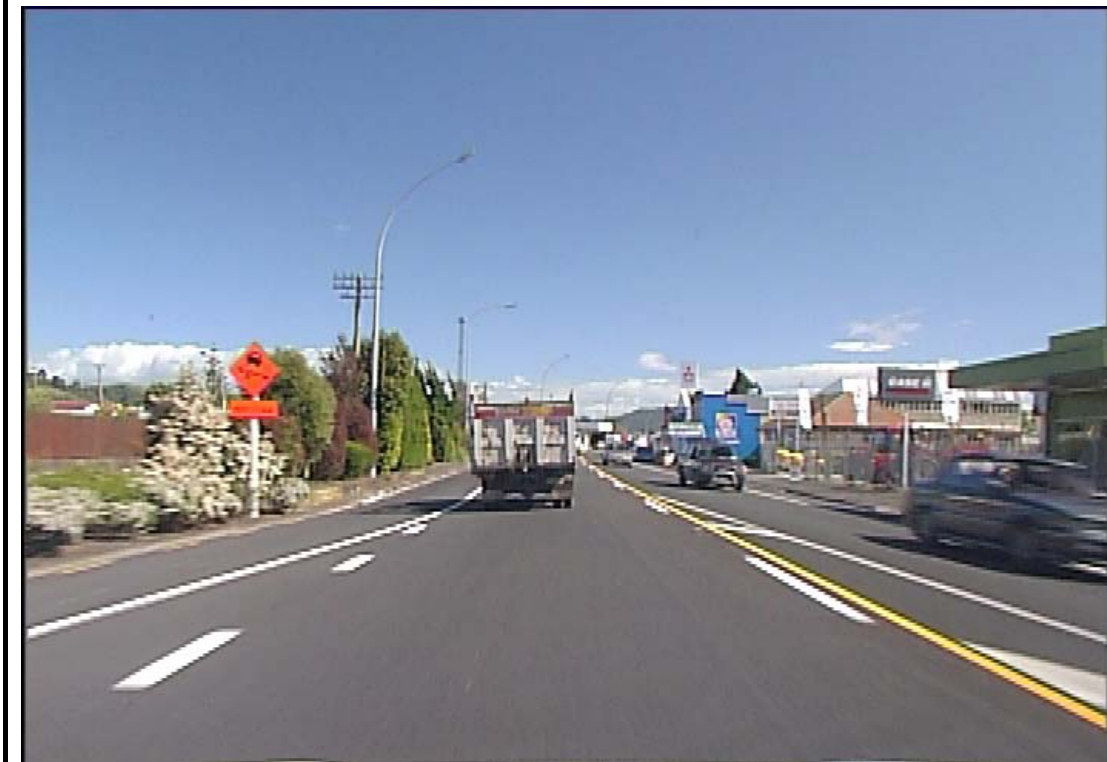
Example 14. TW4 temporary red..
