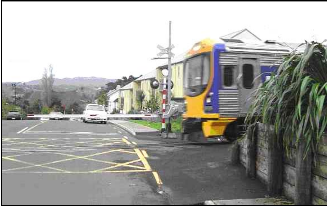
Figure 2.12 An at-grade rail/pedestrian crossing with poor pedestrian facilities.
