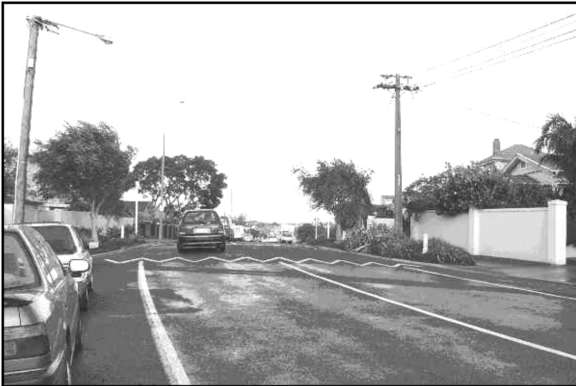
Figure 2.9 Flat-top road humps (platforms).
