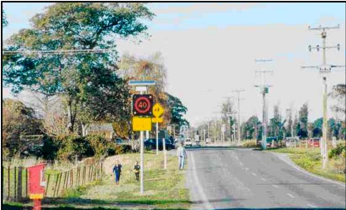
Figure 2.13 School zone signs in operation outside Fairhall School, Blenheim, as an example of an advance automated warning device. NB footpaths should also be provided.
