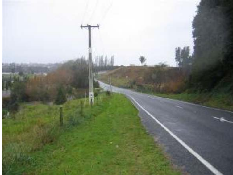
Figure 3.8: Photograph of a poorly designed piece of road.
