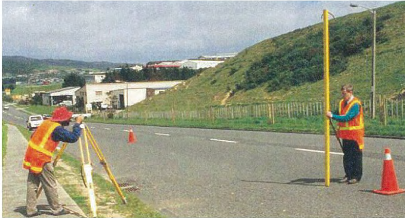
Figure 4.1 Rod and Level Road Profiling.
