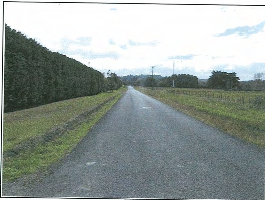
Figure 5.3 General view of Bristol Road test site, looking north.
