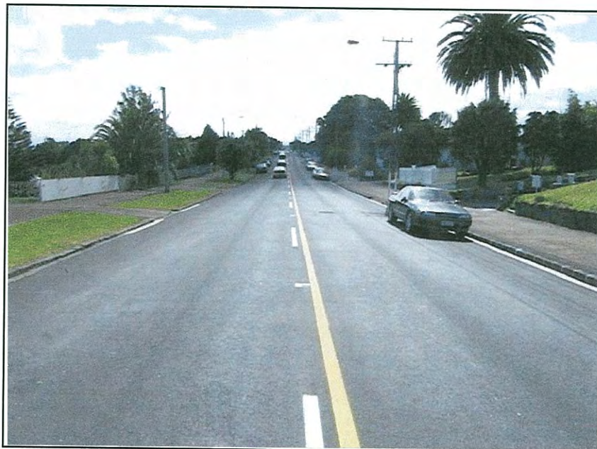
Figure 5.2 General view of Blockhouse Bay Road test site, looking north.
