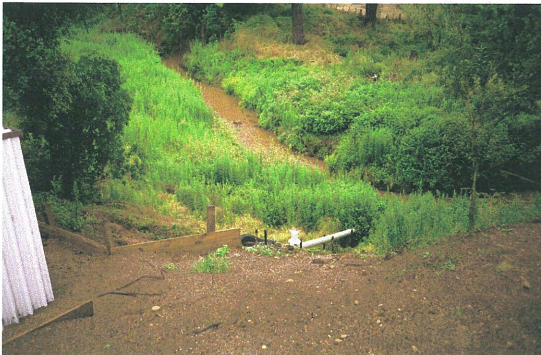
Figure 3.7 Road runoff being piped into receiving stream.
