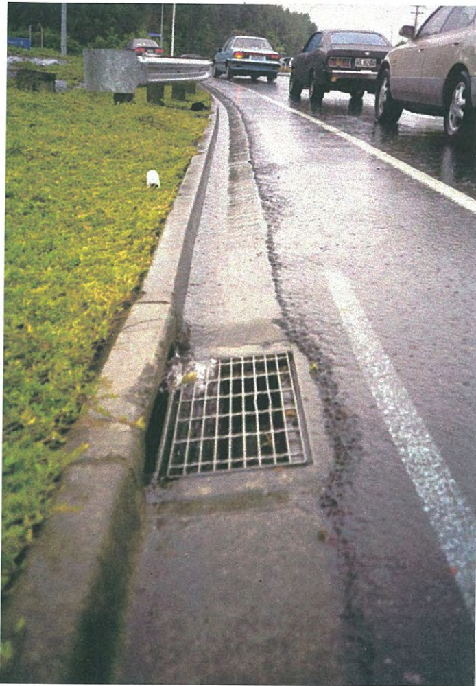
Figure 3.4 The catchpit that received the roundabout runoff.
