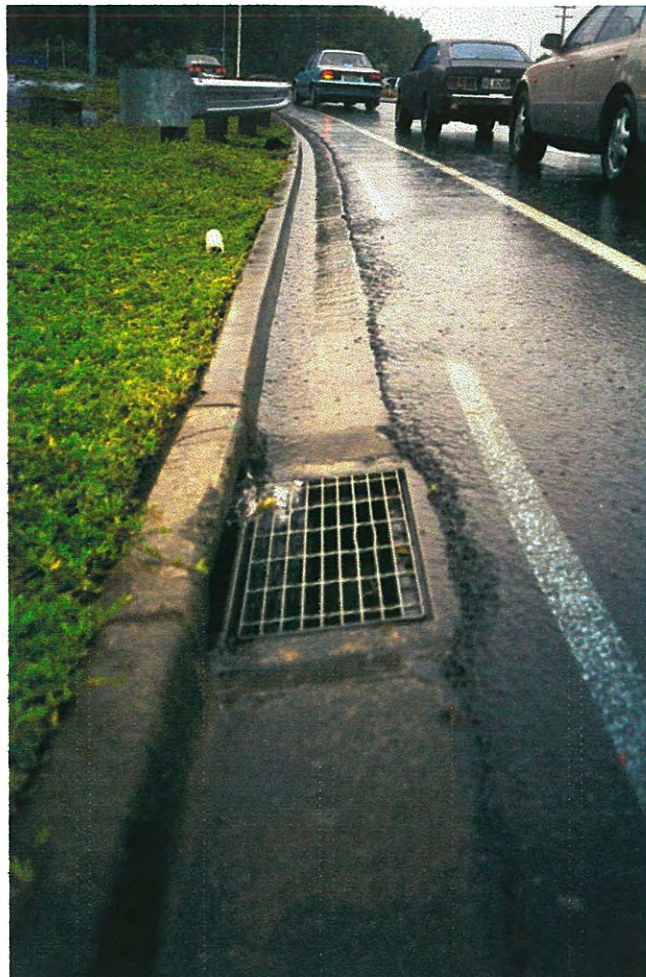
Figure 3.4 The catchpit that received the roundabout runoff.
