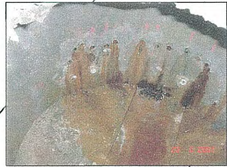
VIEW OF COLLECTION MANHOLE
