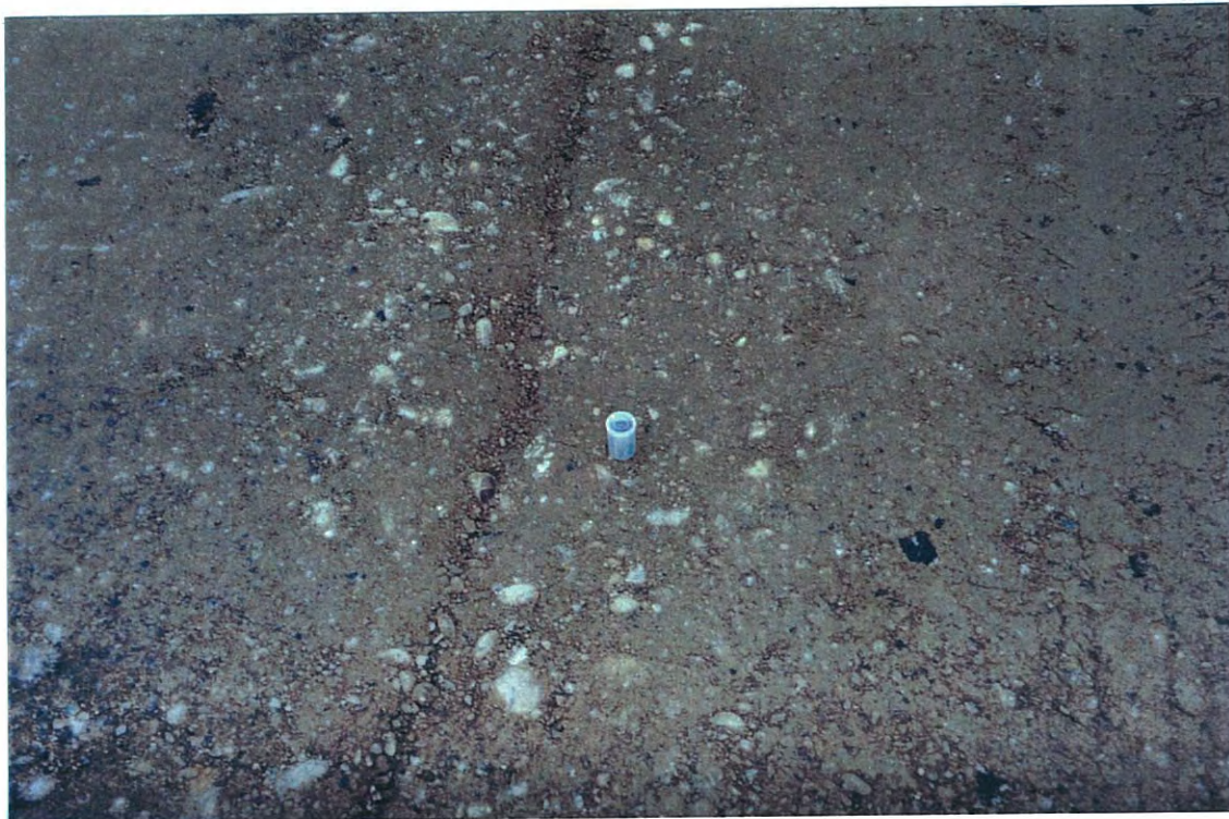
Figure 3-8 Compacted Bitumen Aggregate Mix Prior to Final Shaping
