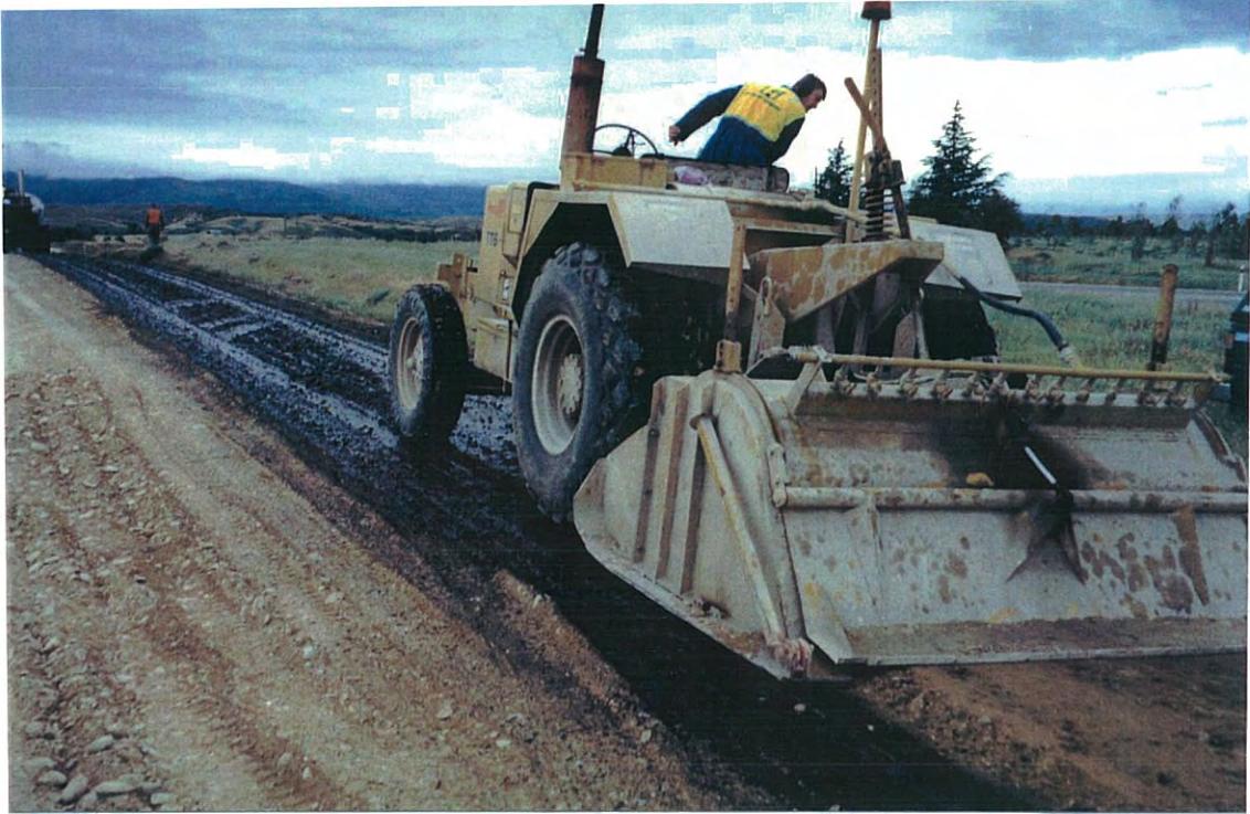
Figure 3-8 Compacted Bitumen Aggregate Mix Prior to Final Shaping
