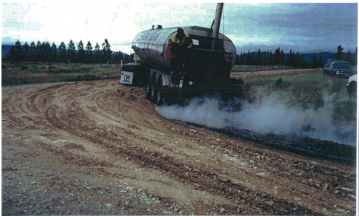
Figure 3-6 Emulsion tanker with purpose built spray bar applying bitumen
