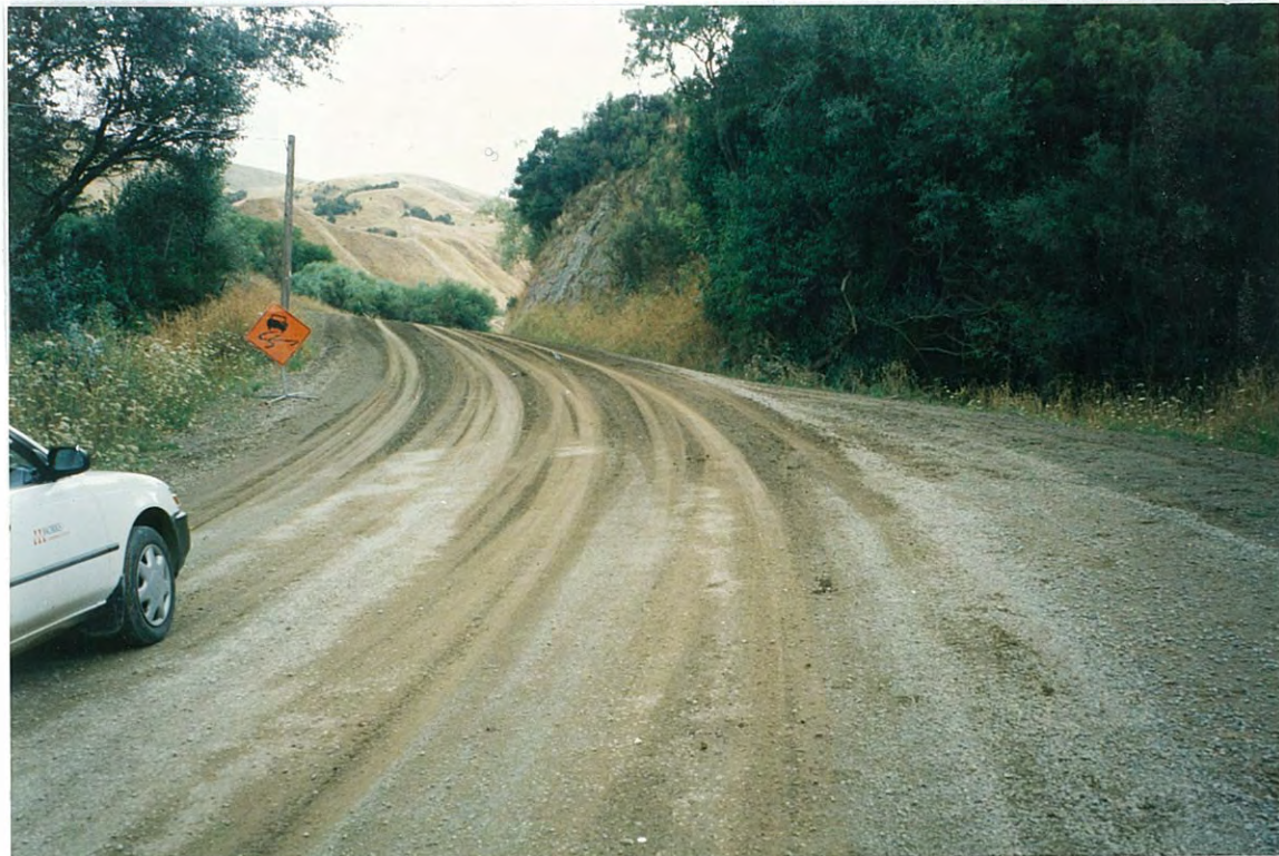
Photo 7 (upper): Section 1 General view of section 1, 1 week following construction. Pavement surface is hard and smooth.
