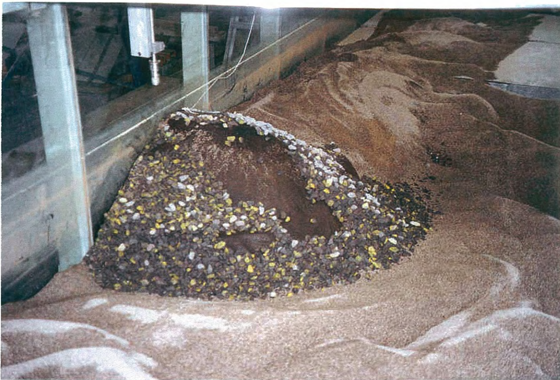
(c) Riprap failure
