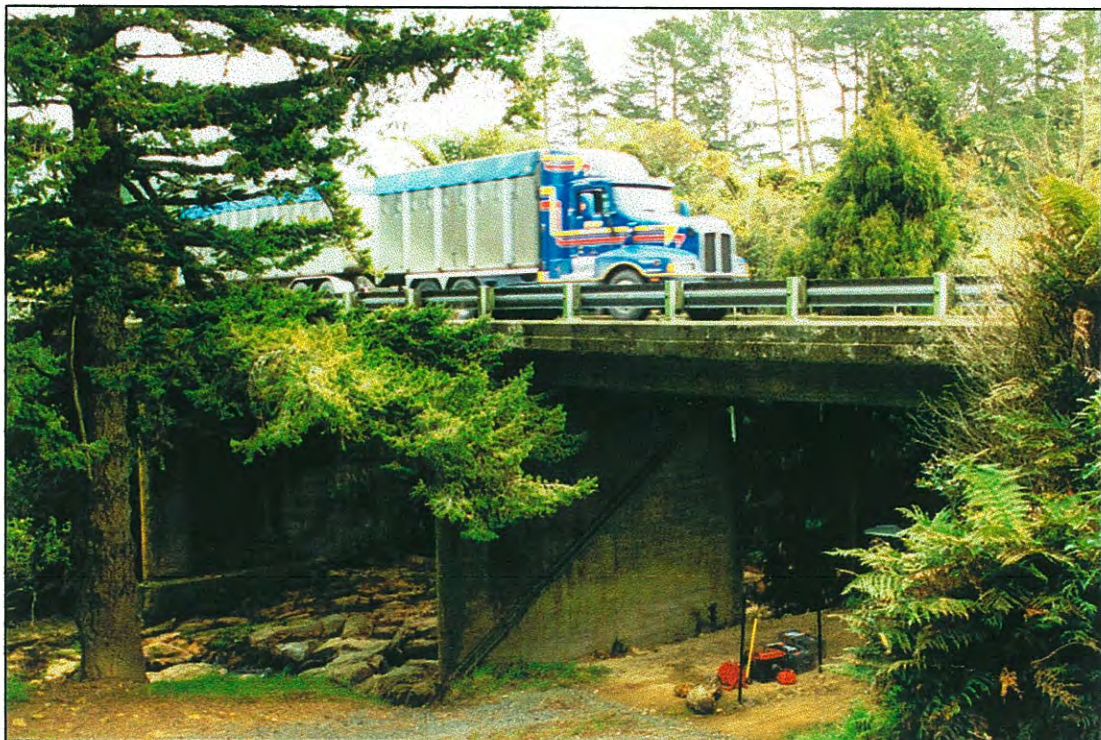
Figure 4.2 The known vehicle used for behavioural testing, on the Tuakopai Bridge.
