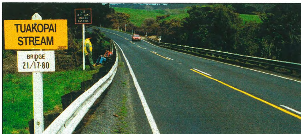
Figure 3.3 Road over the bridge (note the metal guardrail that replaces the original guardrail).
