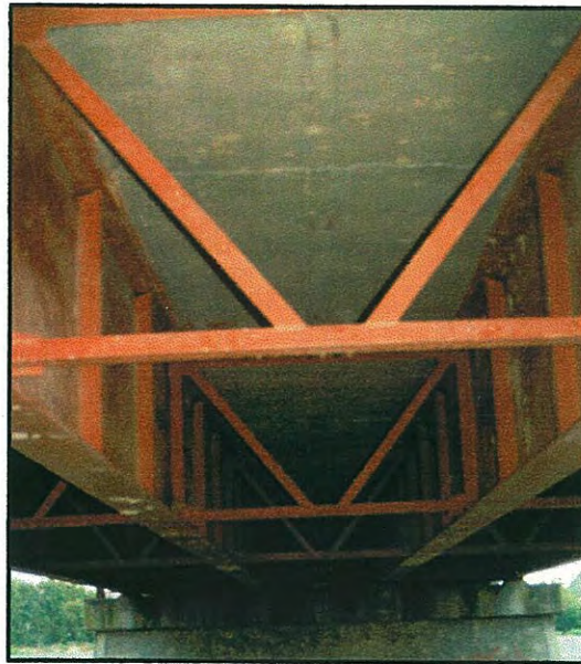
Figure 3.2 Bracing of the main girders.
