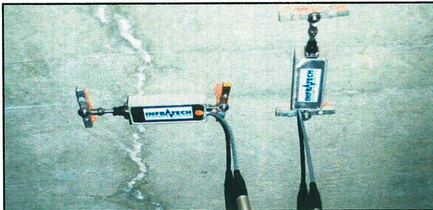
Figure 4.4 Instrumentation on the deck.
