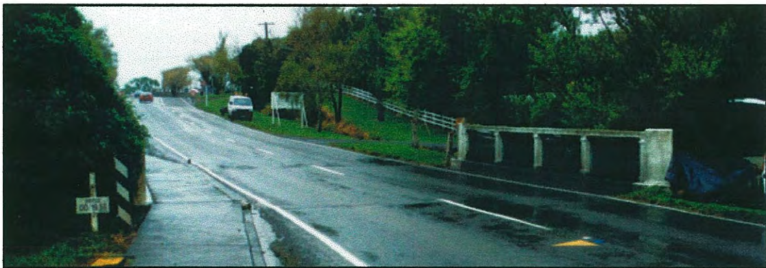
Figure 3.1 Otauru Bridge on SH57 (looking north).
