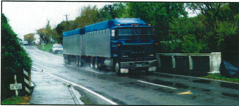
Figure 4.6 The known vehicle on the Otauru Bridge during the behavioural testing.
