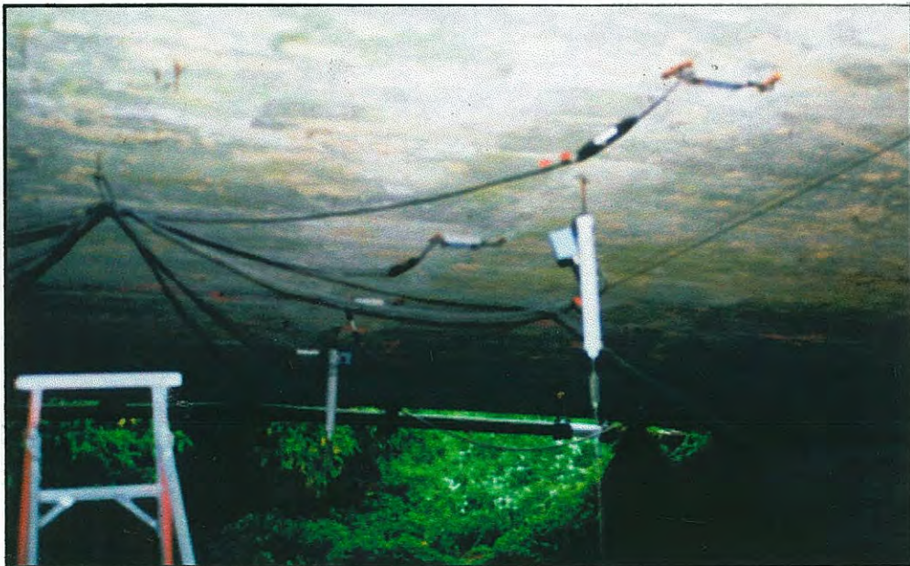
Figure 4.4 Instrumentation installed at the midspan of the slab.
